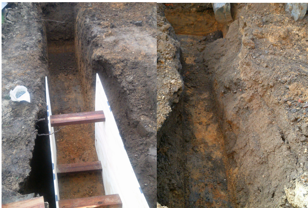
Photographs 1-2 Foundations trenches, looking S
