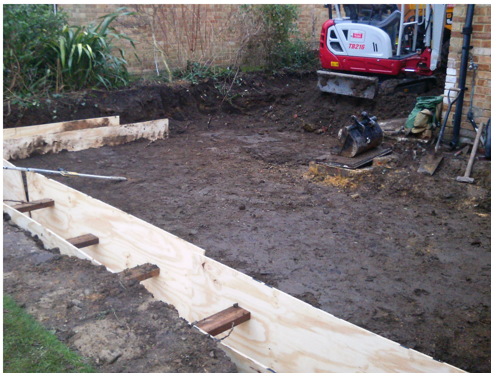
Photograph 3 Foundation trenches and ground reduction, looking SW
