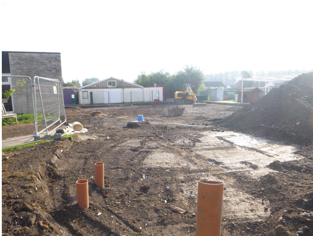
Photograph 4 Strip of first monitoring area down to L5, looking NE
