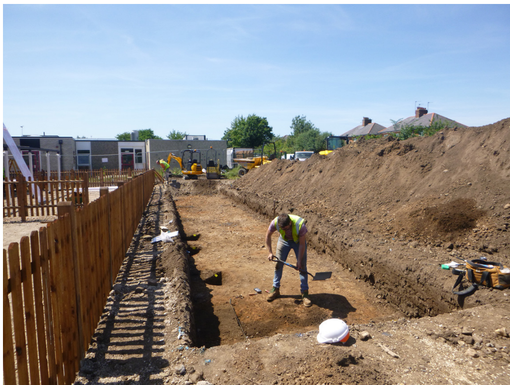
Photograph 5 Excavation of pits in the second monitoring area, looking SW
