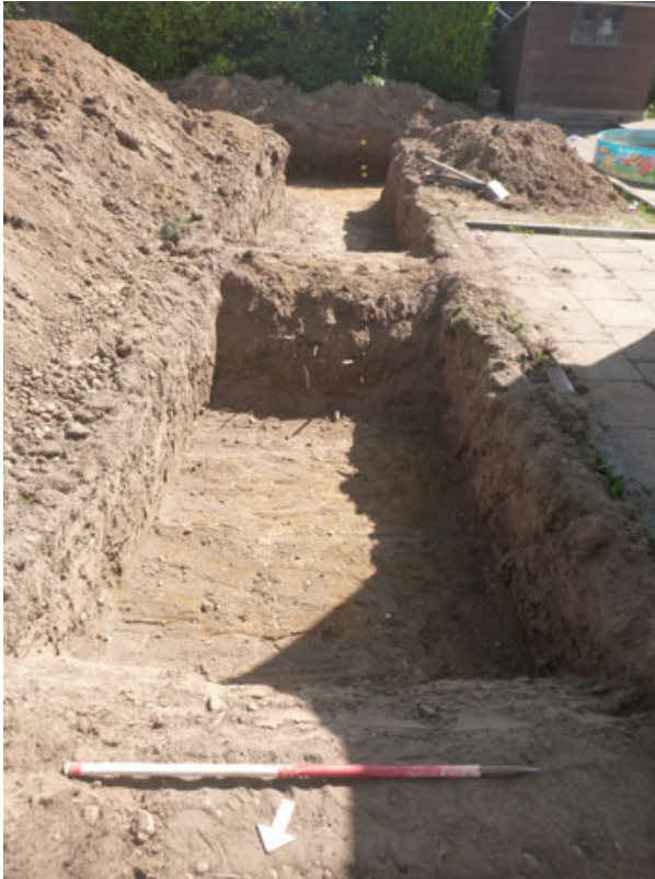
Photograph 3 T3, looking SE
