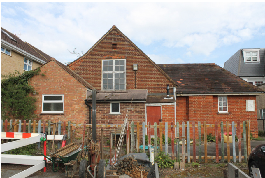
Photograph XII Rear of building, showing all four extensions. Shot taken facing north-east.
