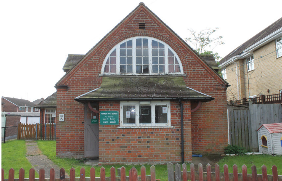
Photograph I Front of building, showing original porch. Shot taken facing south-east.
