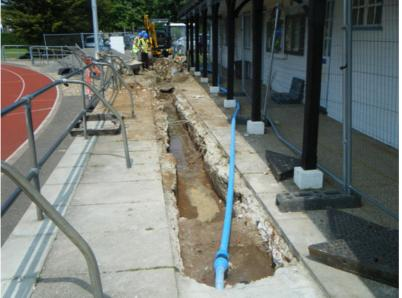
Photograph 1 Main drainage trench, looking N
