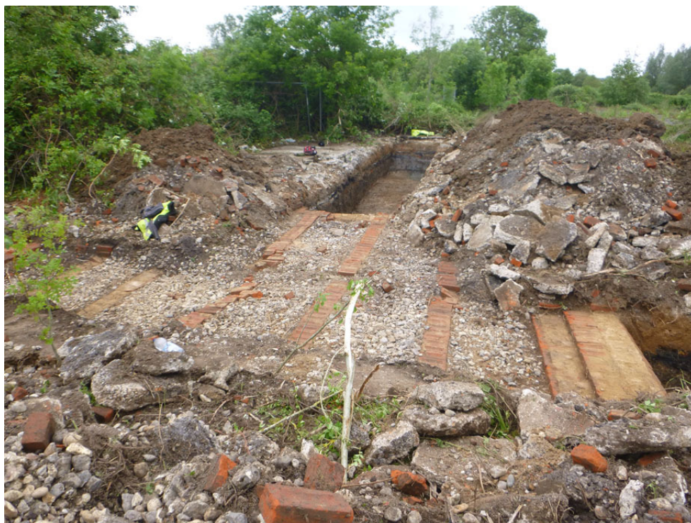
Photograph 5 T2-T3, looking SE
