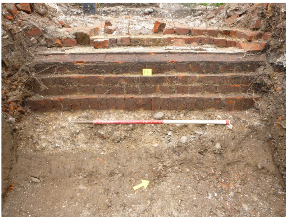
Photograph 11 South-east facing external wall of mill showing low plinth wall with lower moulded chamfered brick course, looking NW
