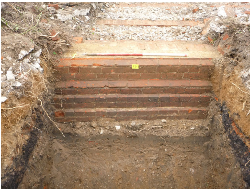
Photograph 6 South-west facing external wall of mill showing low plinth wall with two moulded chamfered brick courses, looking NE
