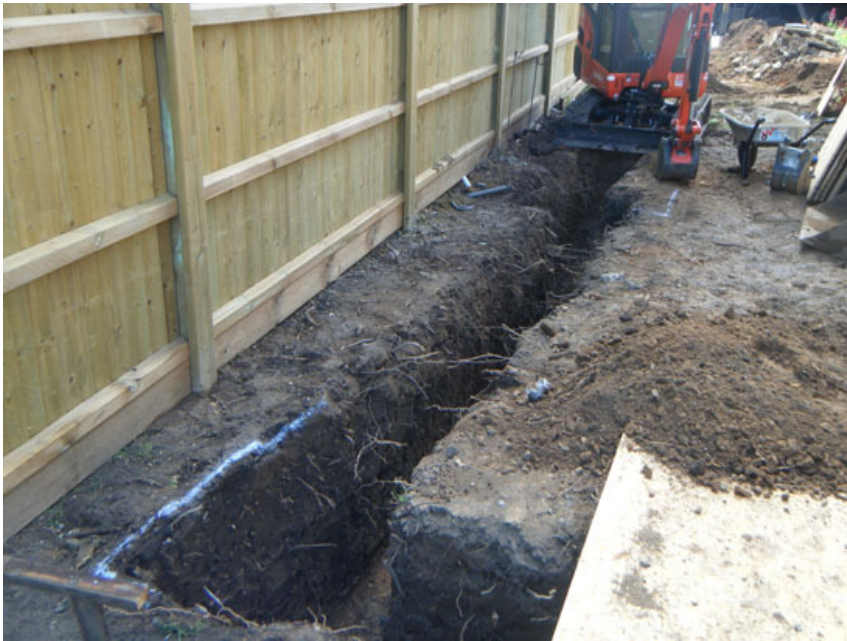
Photograph 1 Foundation trench, looking S
