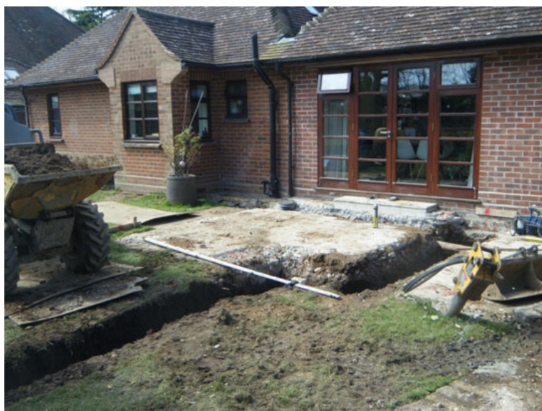
Photograph 1 Rear extension foundation trenches, looking SW
