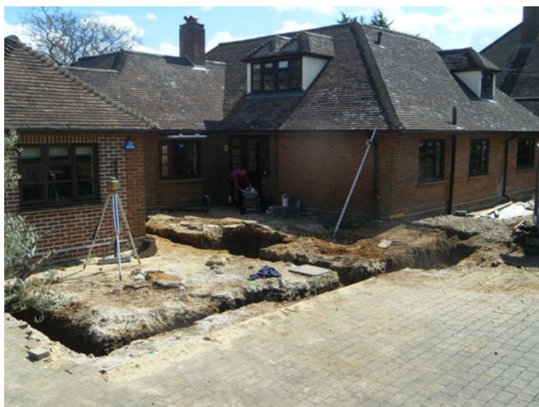
Photograph 2 Side extension foundation trenches, looking NE
