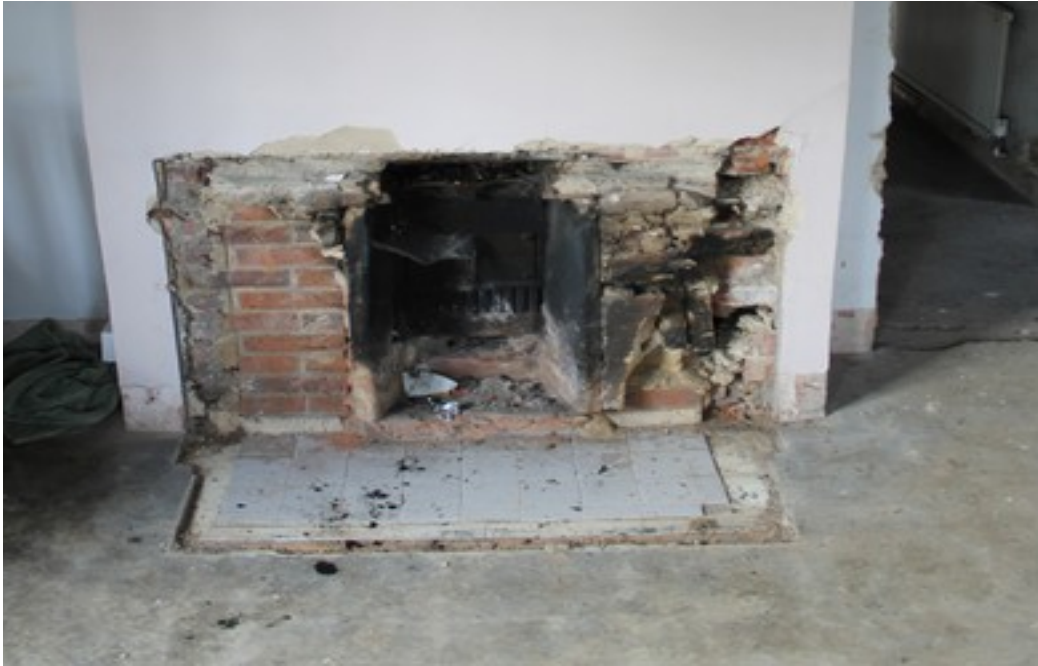
Plate 11 Fireplace in Room 1 with mid 20th-century grill and back boiler inserted – view west.
