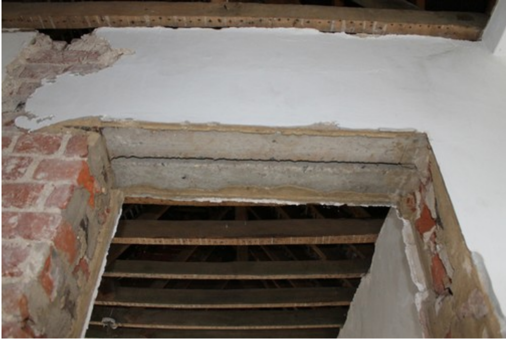
Plate 13 Inserted doorway between Room 2 and 3. Concrete lintel and truncated bricks clearly visible – view south.
