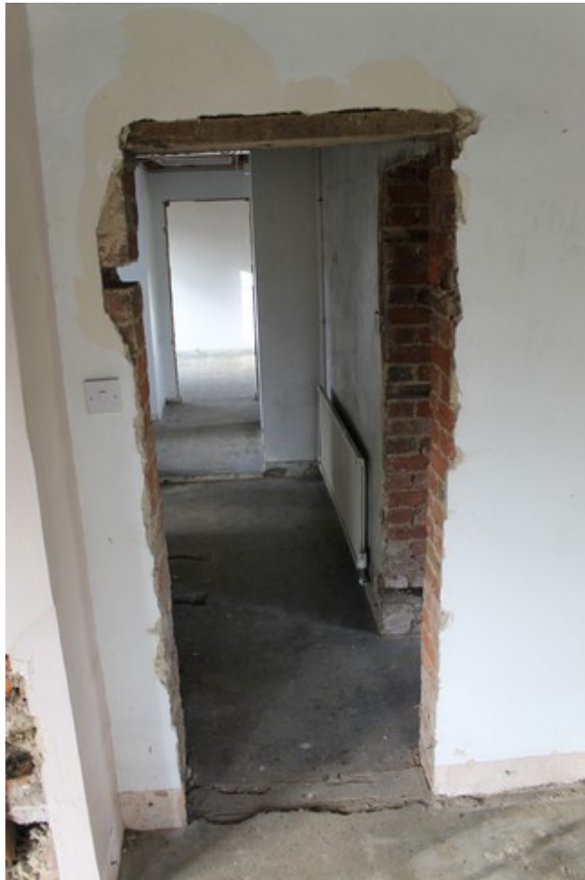
Plate 14 Original doorway between Rooms 1 and 3. Wooden lintel visible – view west.
