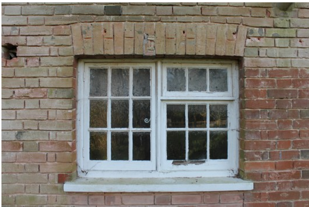
Plate 3 Replacement casement/fly window in north gable end of original lodge. Repaired and damaged arch visible – view south.
