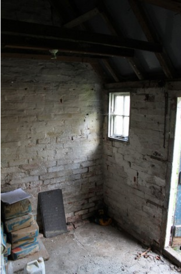
Plate 17 Interior shot of outbuilding – view north-east.
