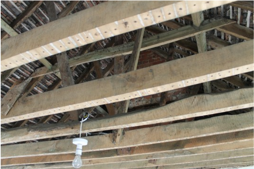
Plate 21 Roof trusses above Room 1, staggered inclined queen posts and collar visible – view south-west.
