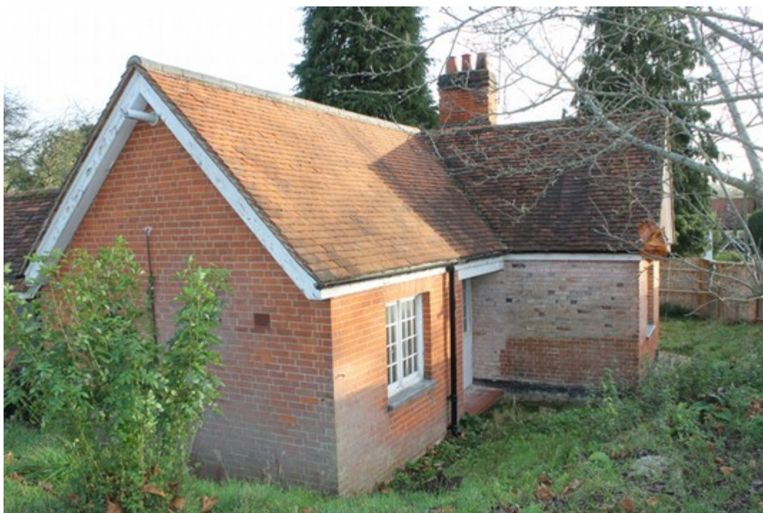
Plate 1 West elevation with 20th century extension in foreground - view north-east.
