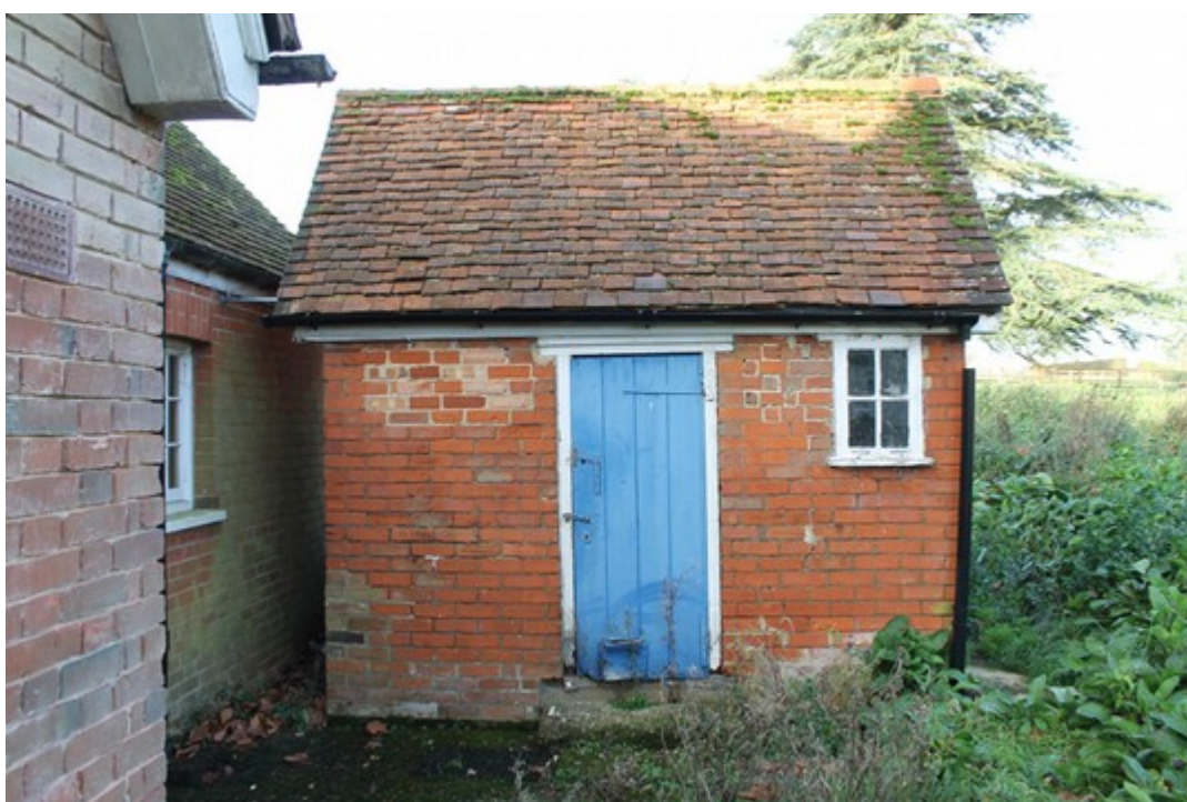
Plate 4 East elevation of the outbuilding – view west.
