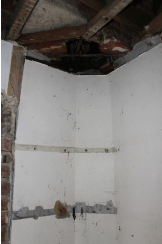
Plate 15 Location of removed fireplace in Room 3. Flue up to chimney visible – view south-east.
