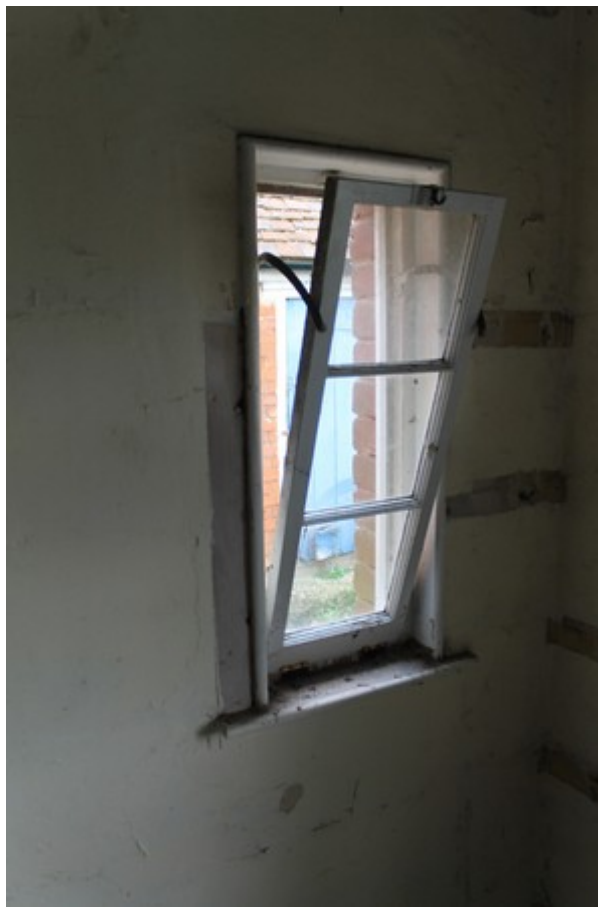
Plate 8 Mid 20th-century hopper window in Room 3 – view north-west.
