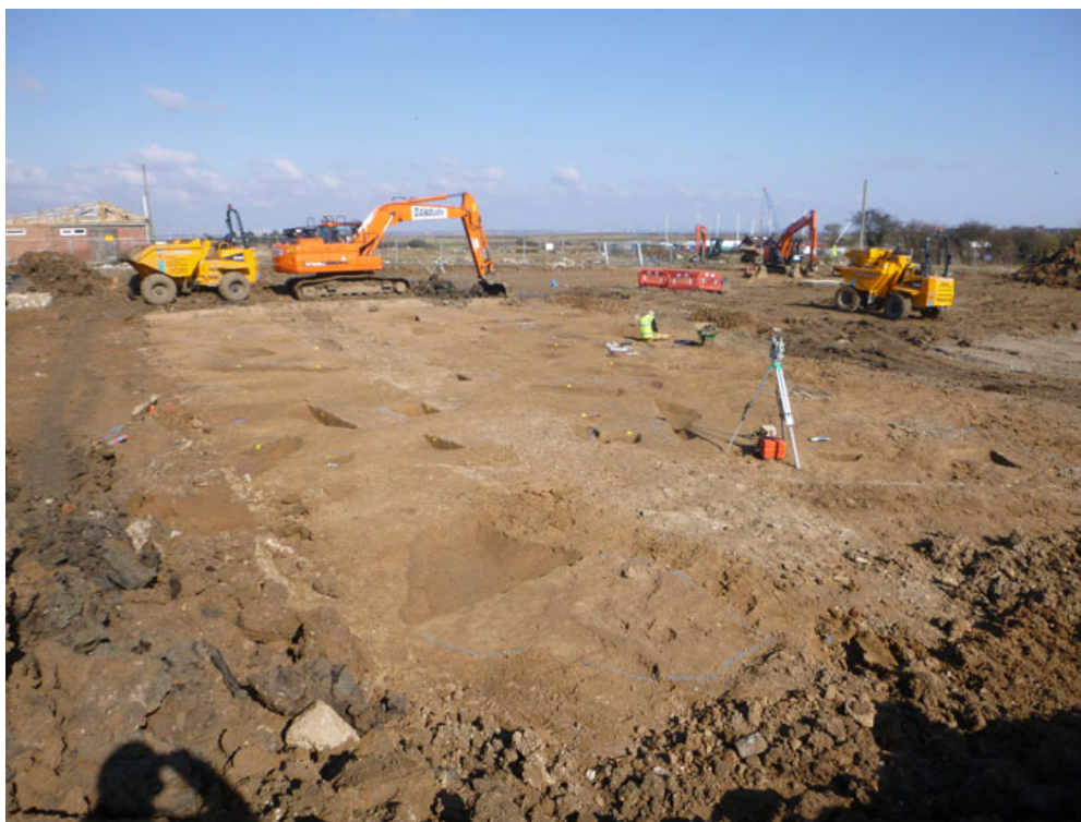
Photograph 2 Excavation area, looking NE
