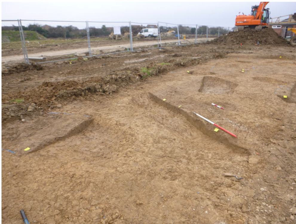
Photograph 1 Excavation area, looking NW
