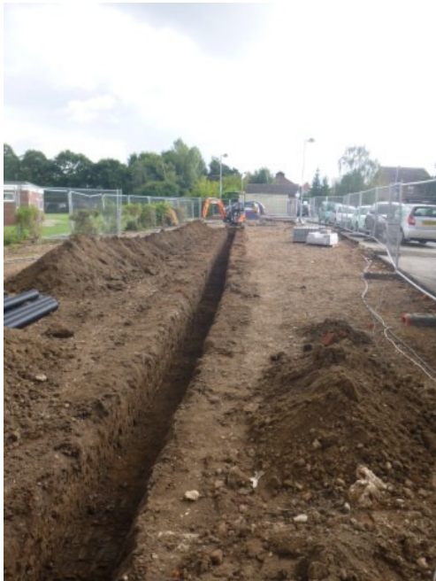
Photograph 5 Electricity trench, looking E
