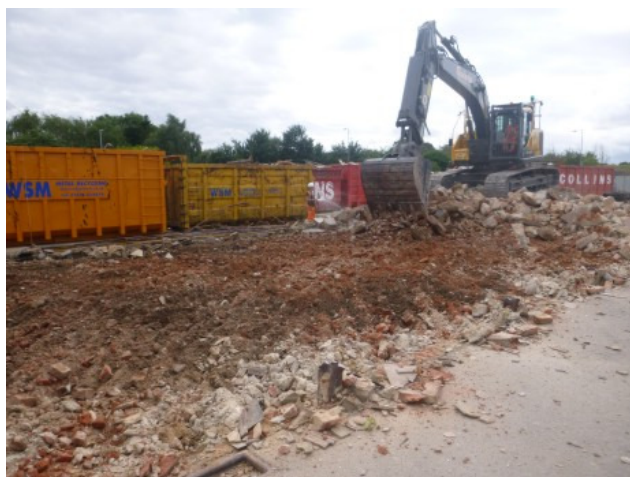
Photograph 1 Slab clearance, looking SW
