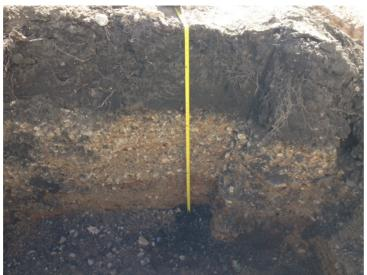
Photograph 5 Section through road surface F1
