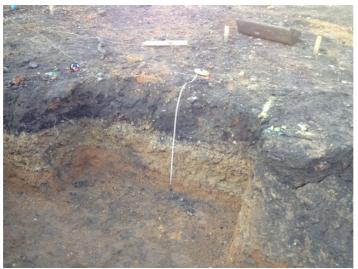
Photograph 6 Section through road surface F1
