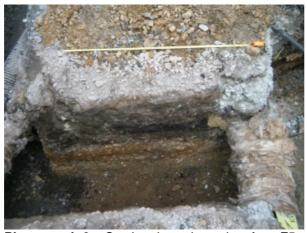
Photograph 9 Section through road surface F5
