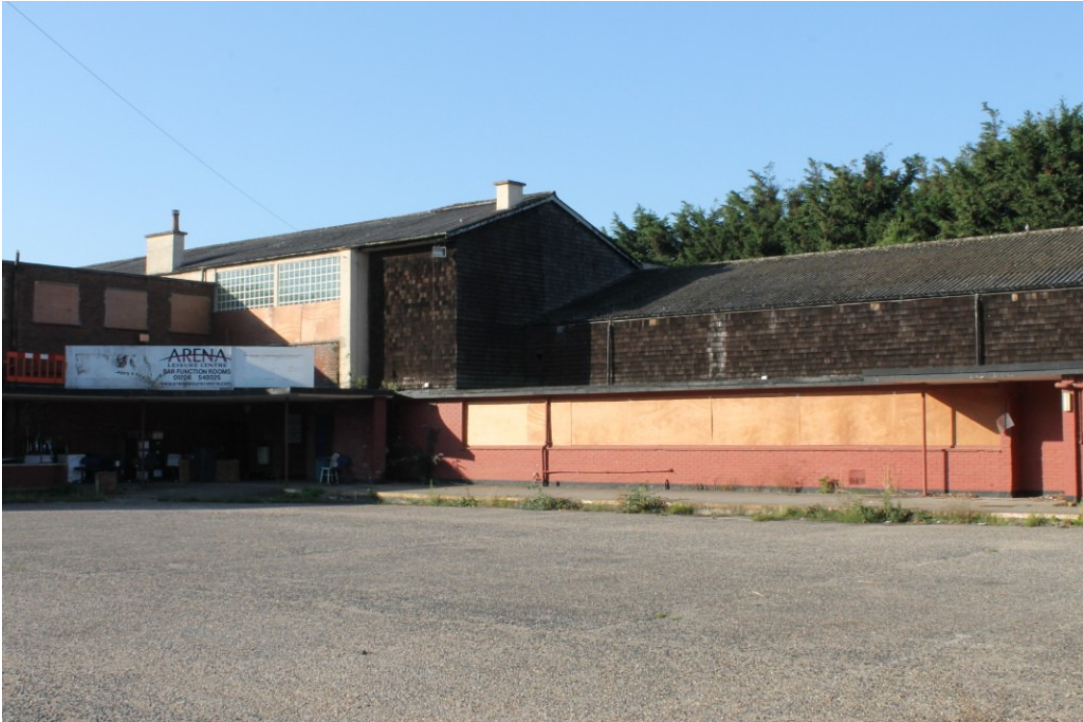
Photograph 3 Northern end of the main range with shingle-clad sides and the reduced central section (formerly three storeys) – view south
