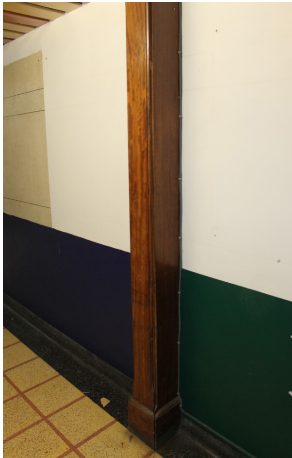
Photograph 15 One of the steel supporting posts of the building's superstructure encased in timber veneers, located in GF2. The original flooring and wall covering can also be seen – view south
