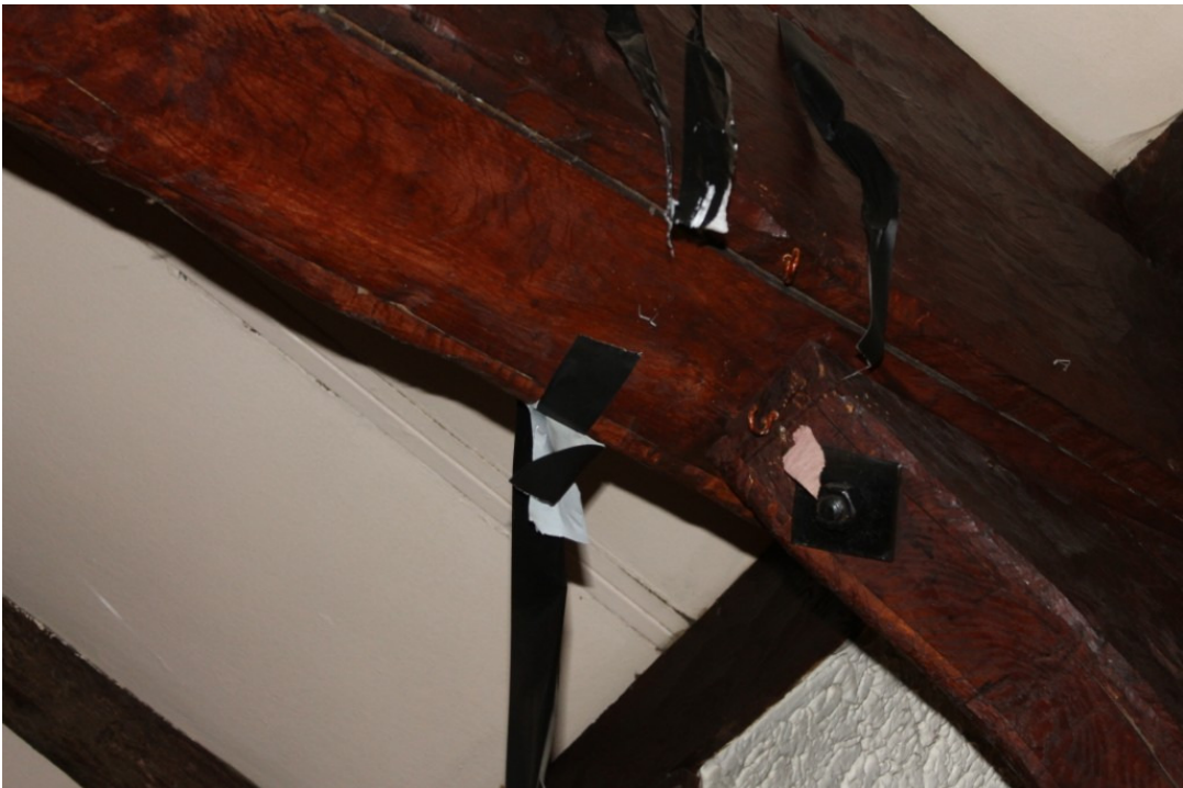
Photograph 28 Tie beam and brace of truss in FF1, showing timber veneers attached to steel superstructure
