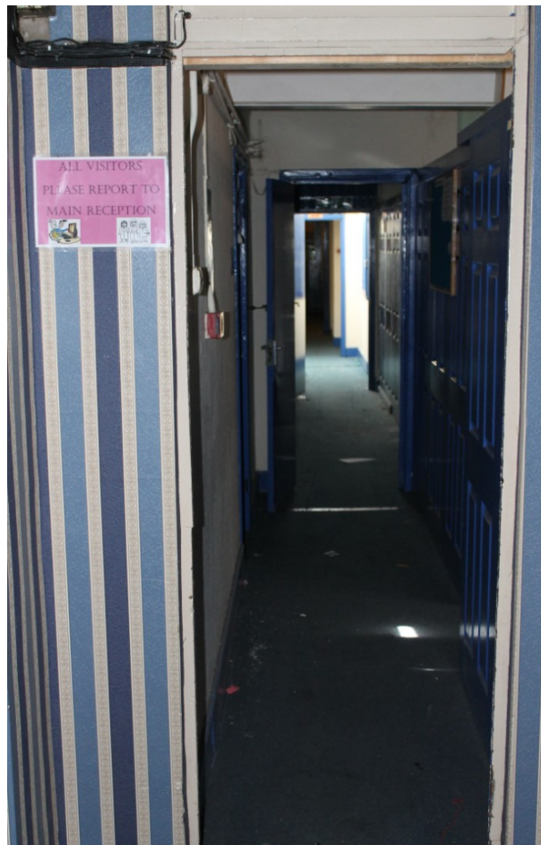
Photograph 32 Doorway providing access to FF3 – view north-east
