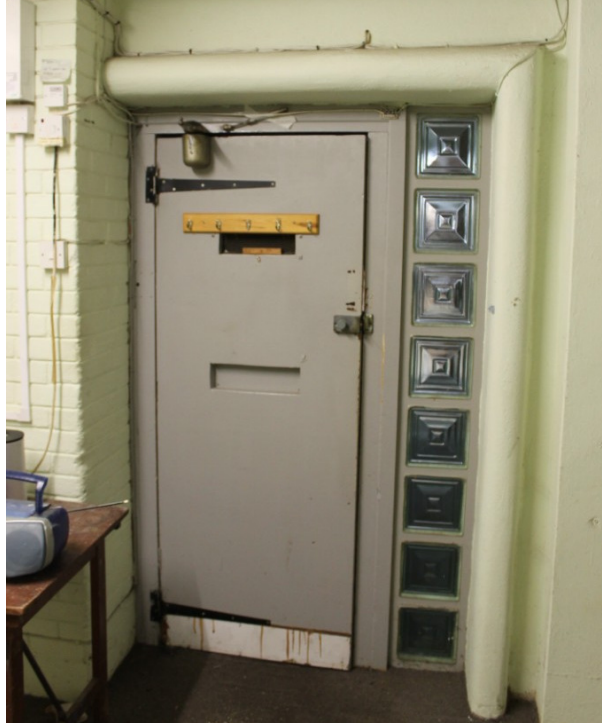
Photograph 13 A second original entrance to the NAAFI located in GF2 – view south
