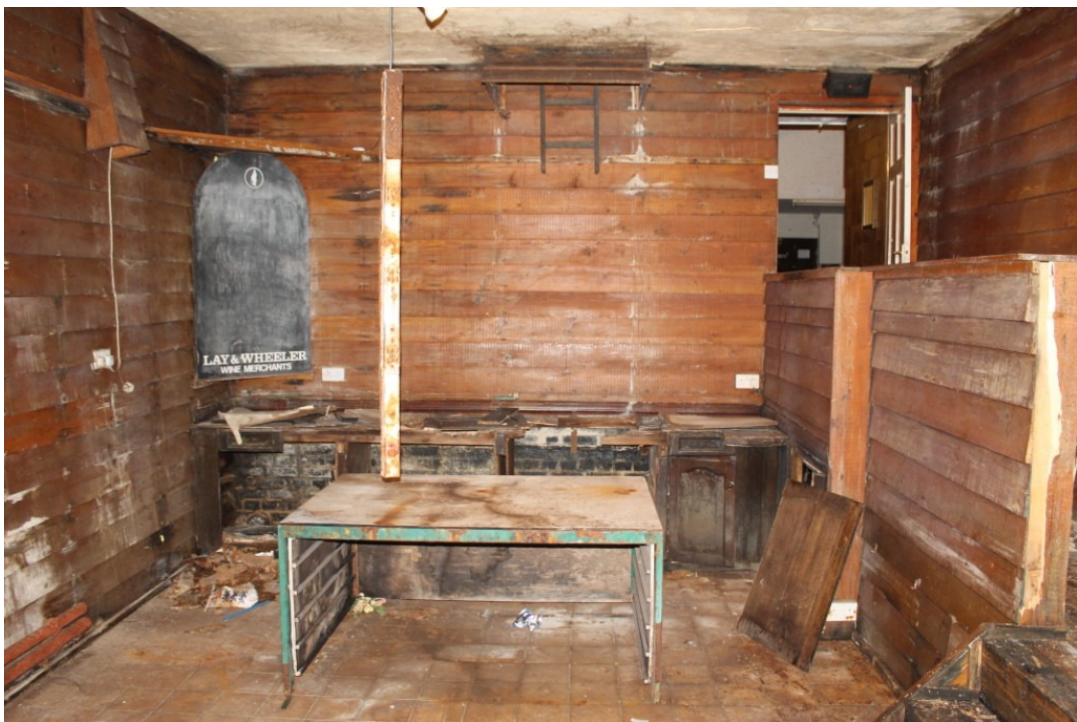
Photograph 22 Auxiliary bar/games room 'k' located in GF3 - view north
