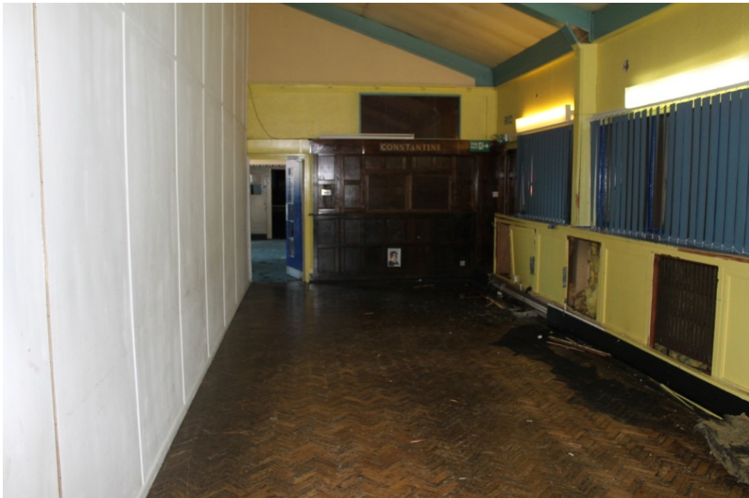
Photograph 29 Western half of FF2 showing the original bar, parquet flooring and inserted stud wall to the left – view south-east
