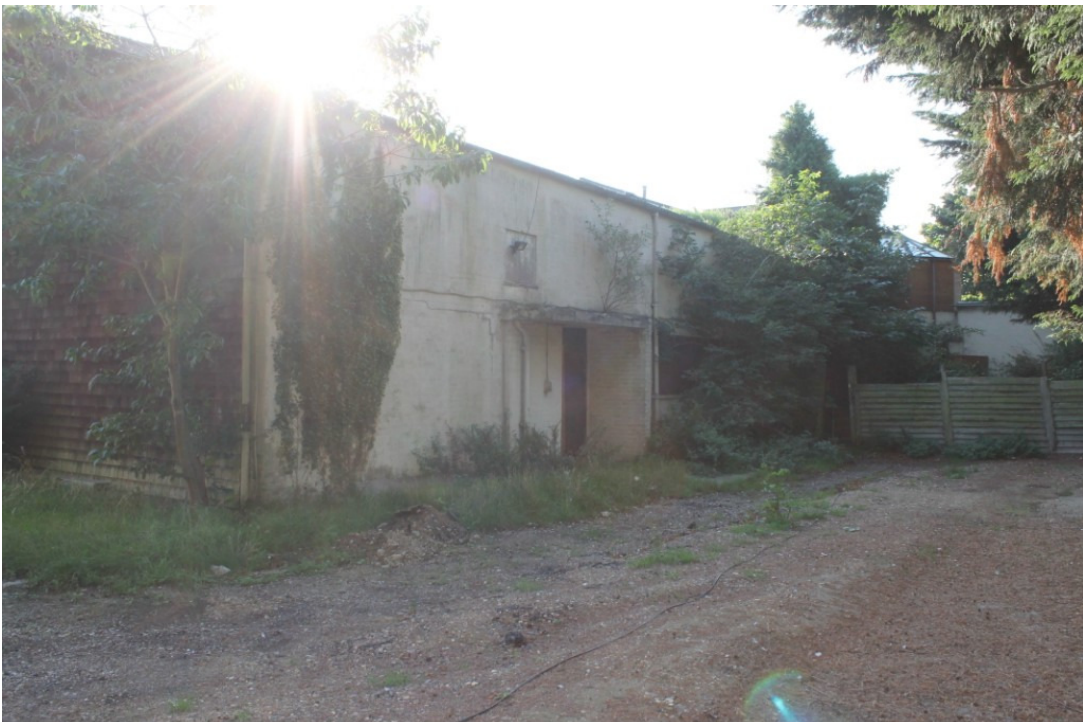
Photograph 4 North-west elevation of GF1 with GF6 in the background – view south-east
