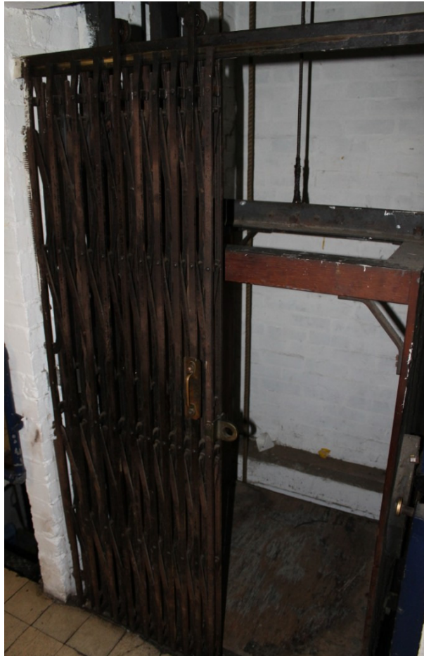
Photograph 20 Mechanized barrel hoist to the cellar below GF3 – view west
