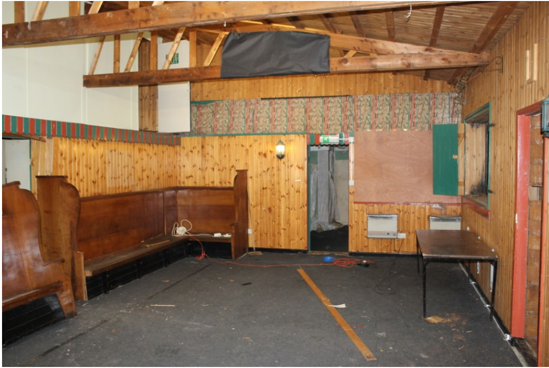
Photograph 21 Auxiliary bar/games room 'j' located in GF3 - view south-east
