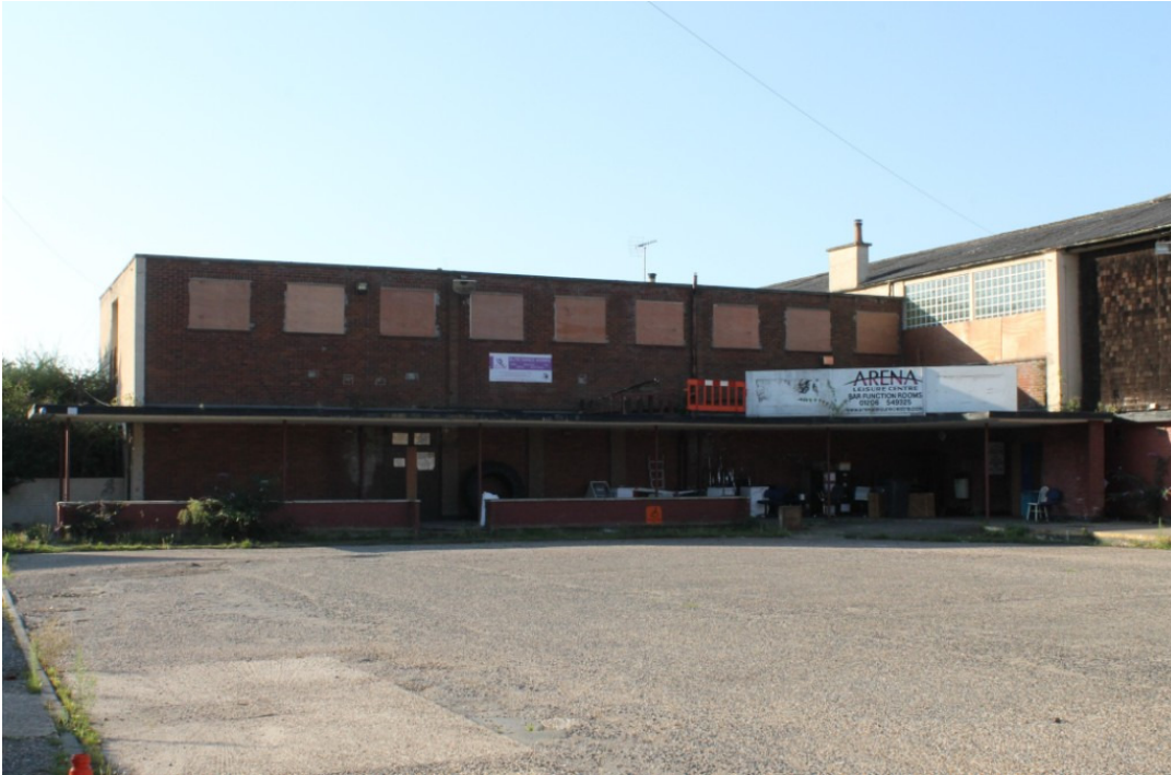
Photograph 2 Two-storey extension on the east side of the Arena (GF3 and FF3) with the gabled main range to the right (GF1) – view south
