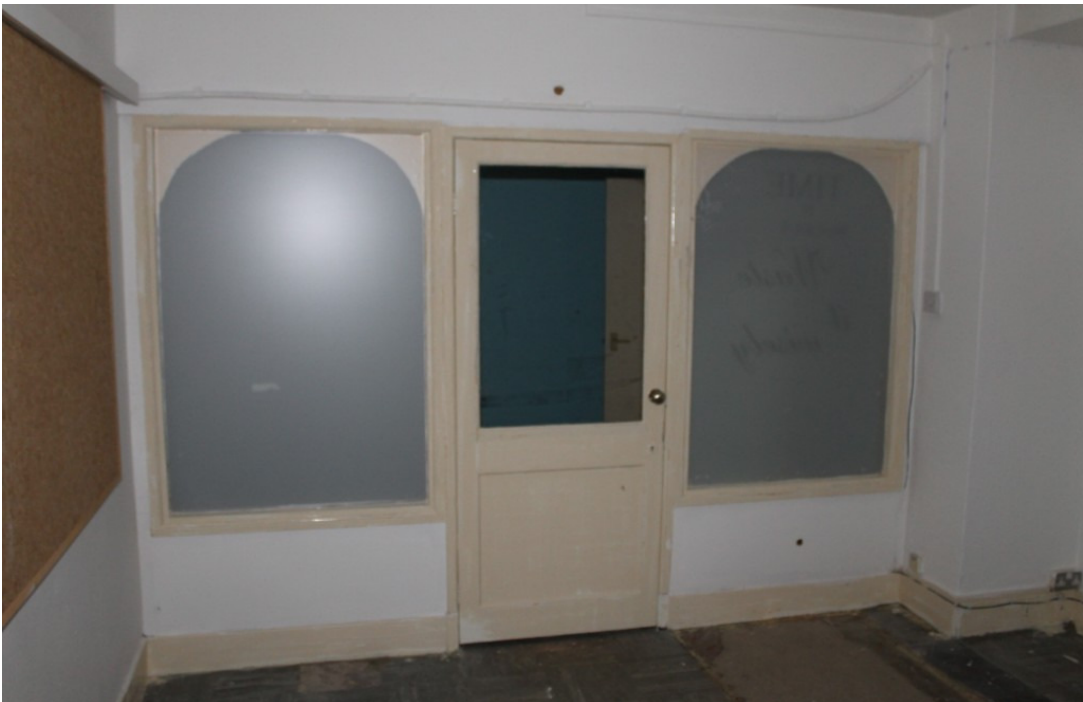
Photograph 11 Interior view of a plate glass shop front, located at the south end of GF1 – view east
