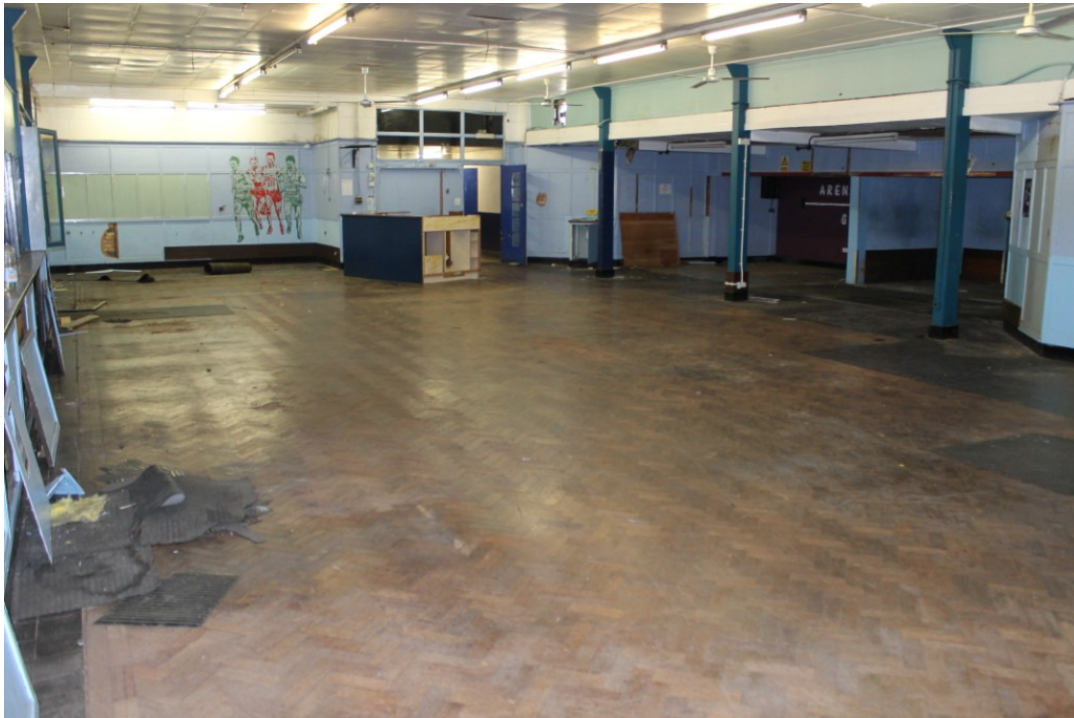
Photograph 23 The Arena Gym, located in GF4, with the original parquet flooring and tiled border - view north
