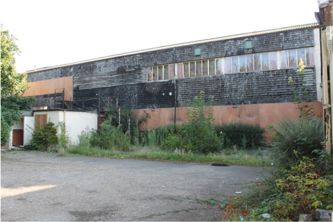
Photograph 7 South-east elevation of GF2 and FF2/FF1 – view north-east
