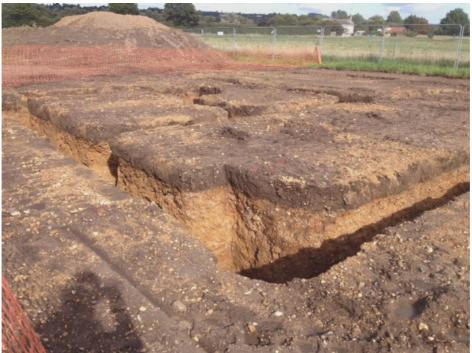
Plate 6: plot 1 footings, showing typical soil profile.
