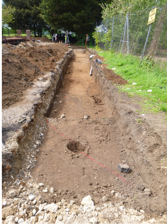
Plate I T1 long shot. View facing south-west. Modern services present in foreground.
