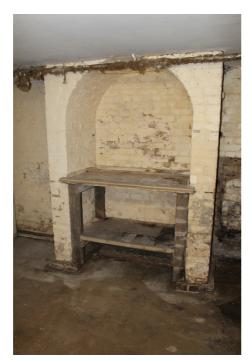
Plate 8 Original brick alcove in basement of Spurrier's House – view south-east
