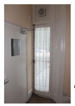
Plate 5 Original French doors of Spurrier's House truncated by inserted stud wall - view north-west
