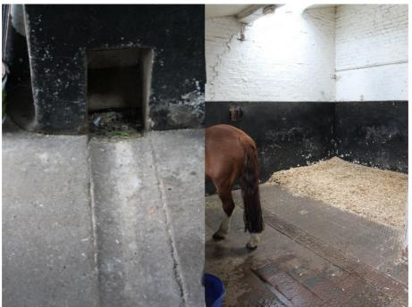
Plate 22 Original drainage gullies and floor surface in the former Spurrier's House stable block
