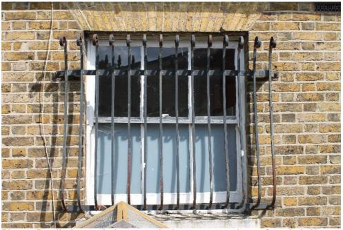
Plate 3 Detail of wrought iron security bars on extension to Spurrier's House - view north-west
