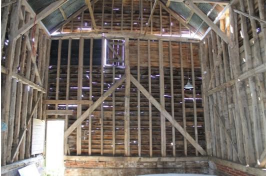
Plate 8 The south-west frame, rebuilt after collapse, with modern machine-cut studs and nailed plank bracing – view south-west
