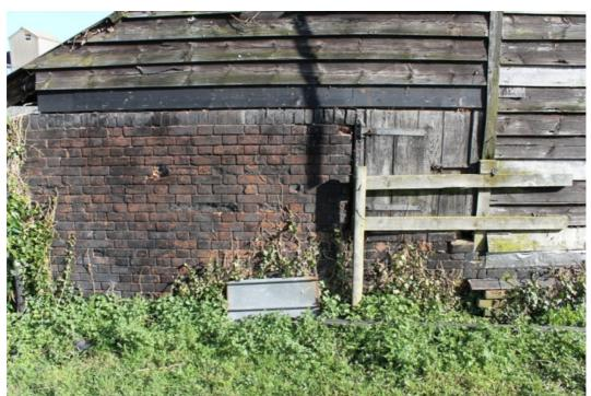
Plate 4 South-west elevation of the lean-to, with Flemish bonded brickwork and the feed door with hinges identical to those of the stable block - view north-east
