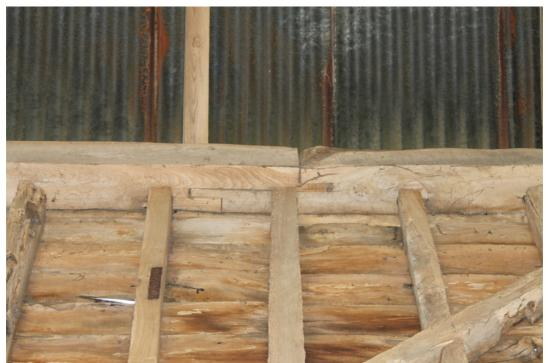
Plate 11 Face-halved scarf joint with bladed abutments, secured by four pegs in the wall plate of bay 5 – view south-east
