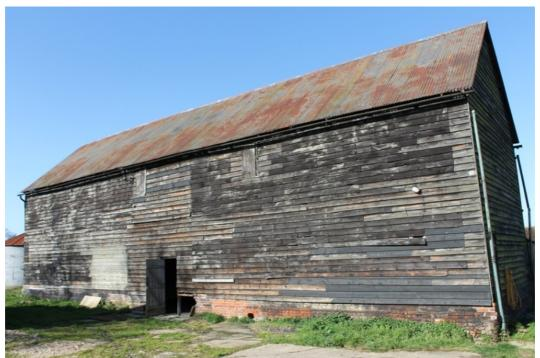
Plate 5 South-east elevation, showing the blocked cart door opening and the inserted pitching doors below the eaves - view south-west
