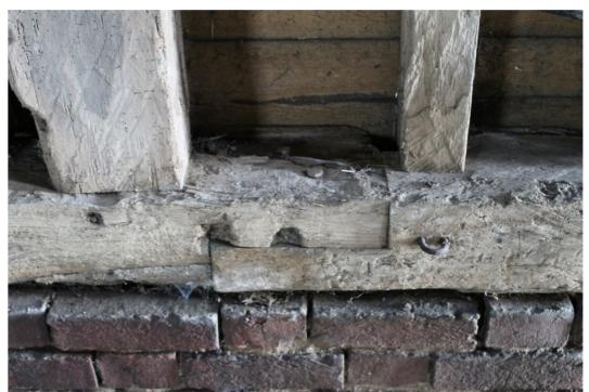
Plate 10 Detail of edge-halved scarf joint, secured by two pegs in the sill beam of bay 6 – view south-east
