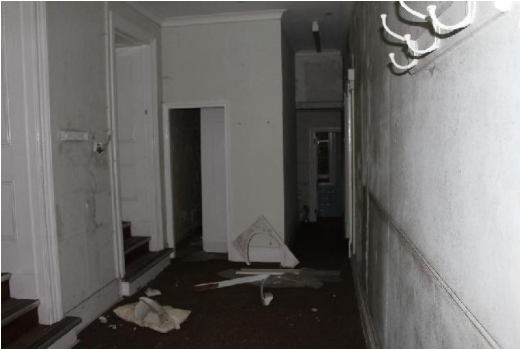
Plate 35 The converted landing of the former stairwell iii , with the inserted shower room, the 1904 ablution block to the rear and the original doorways to the servants' quarters in the left-hand wall – view north-west
