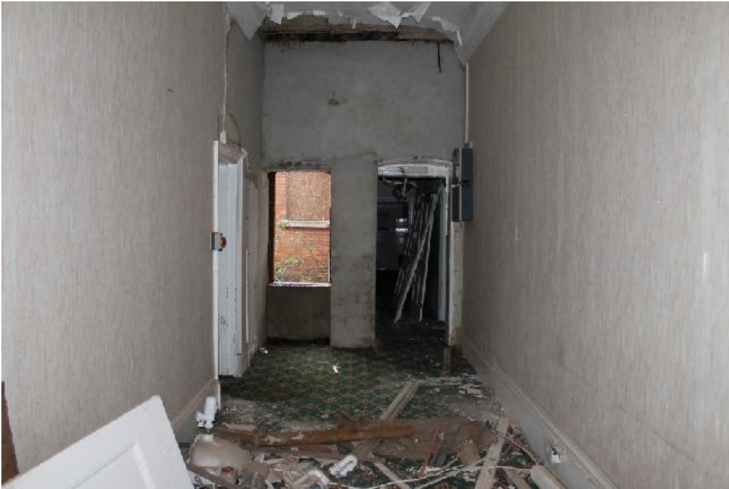
Plate 17 Entrance way iii with the removed staircase and the 1904 toilet block to the rear - view north-west
