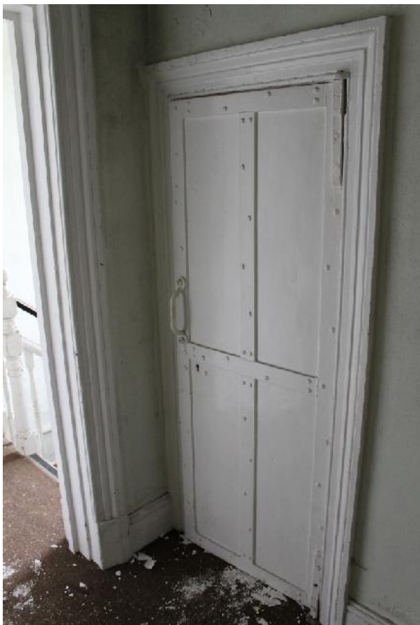
Plate 33 Iron door to strongroom 20, converted from the former servants' quarters for Officers Nos.2 and 3 - view west
