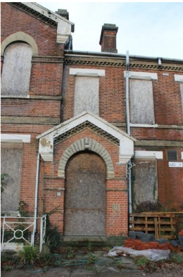
Plate 4 Entrance way iii , showing the projecting gabled porch with the yellow stock brick embellishments, sandstone bell pull and iron bracket for gas lamp – view north-west
