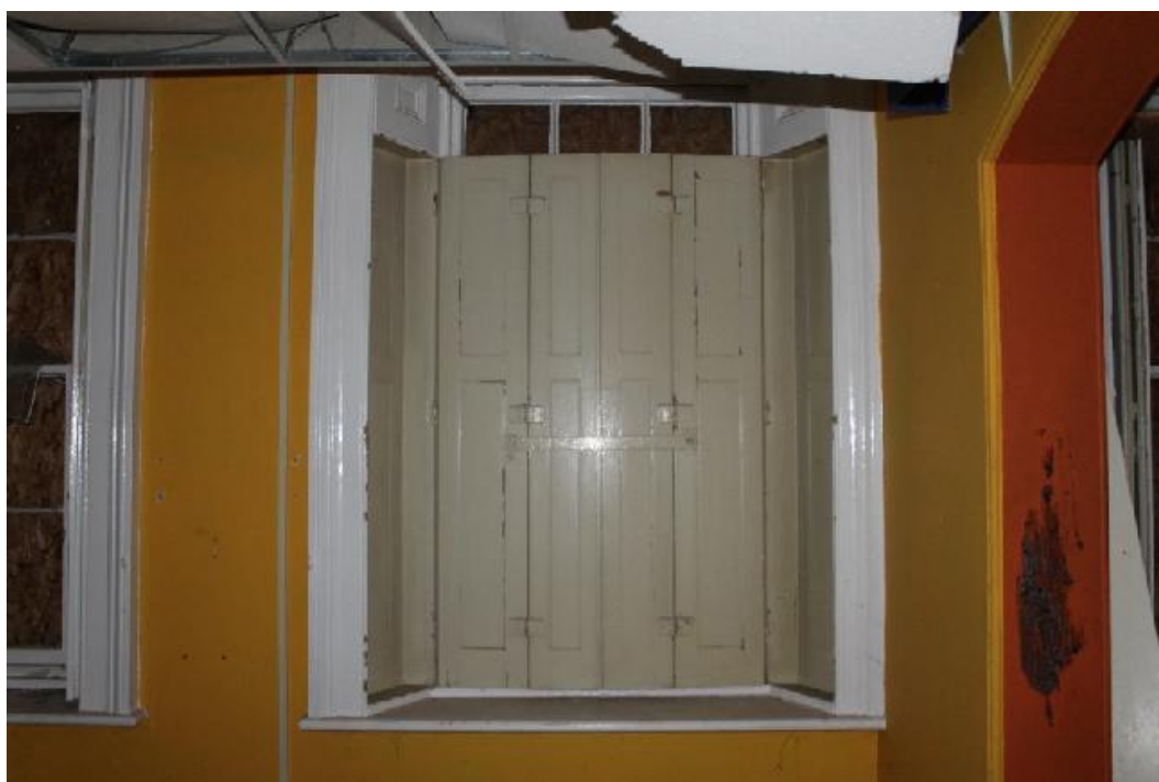
Plate 22 Example of the sash windows with recessed wooden shutters in the ground floor rooms of the 1874-5 building - view south-east
