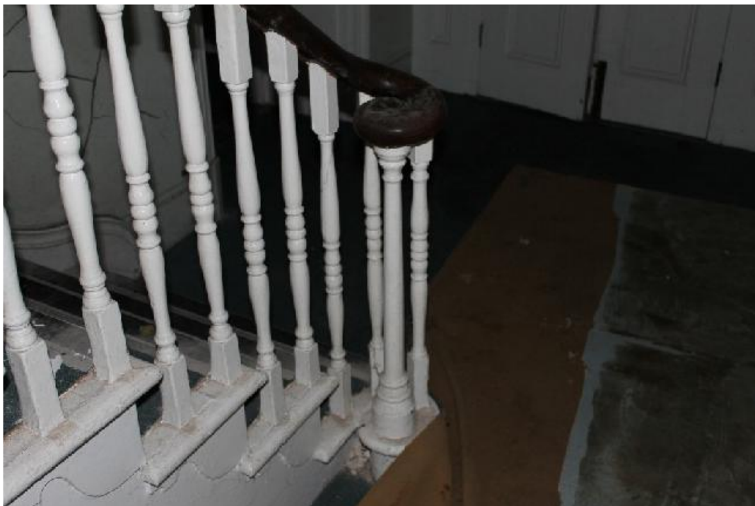
Plate 16 Stairwell iv , detail of the mahogany banister with spiral end and the turned balusters of the open string staircase
