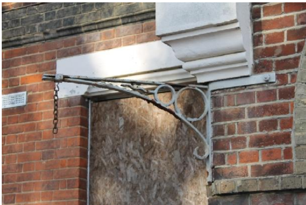
Plate 6 Detail of the iron bracket and chain for the original gas lamp on the corner of entrance way i
