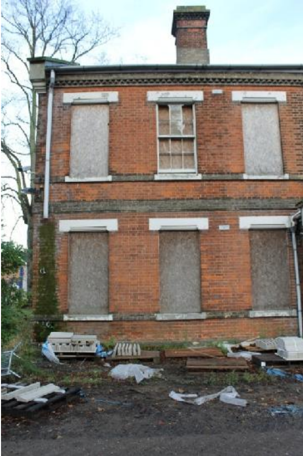
Plate 9 South-east elevation of the 1904 extension to the Officers' Quarters, showing the continuation of the architectural embellishments; the change in the brickwork is visible in the top right of the photograph - view north-west
