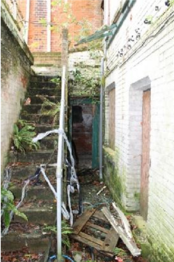
Plate 39 Stairwell vi, leading from the basement kitchen and underground storage area to the yards at the rear of the building: the original coal store is visible at the end of the passage – view north-east
