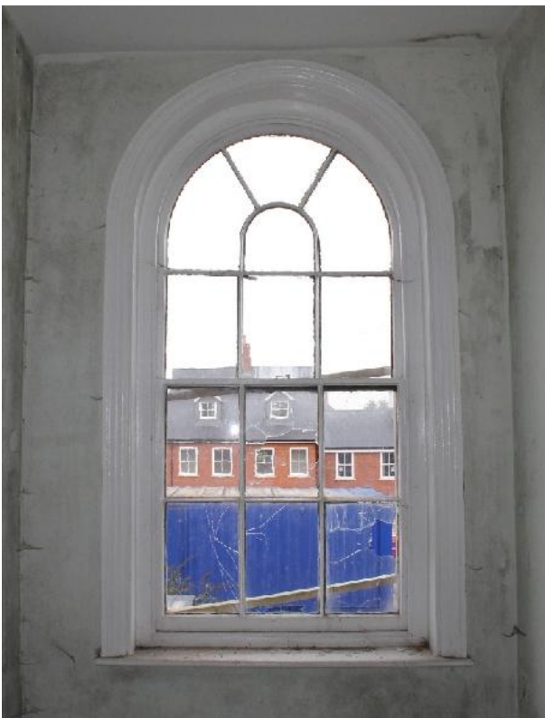
Plate 30 Example of the Italianate sash windows found in rooms 18-21
