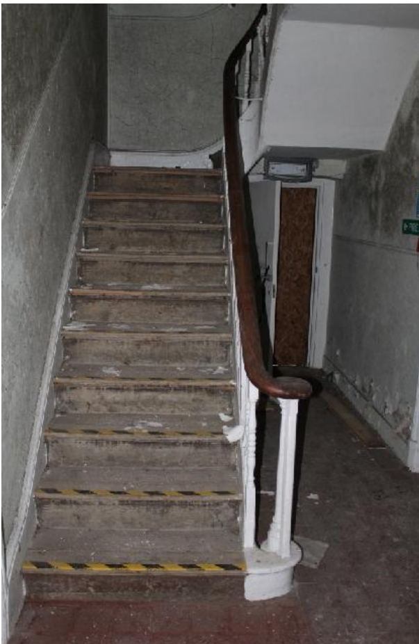
Plate 38 Stairwell v, the basement stairs with the same mahogany banister with spiral end and turned balusters as the staircases of the entrance ways – view north-west
