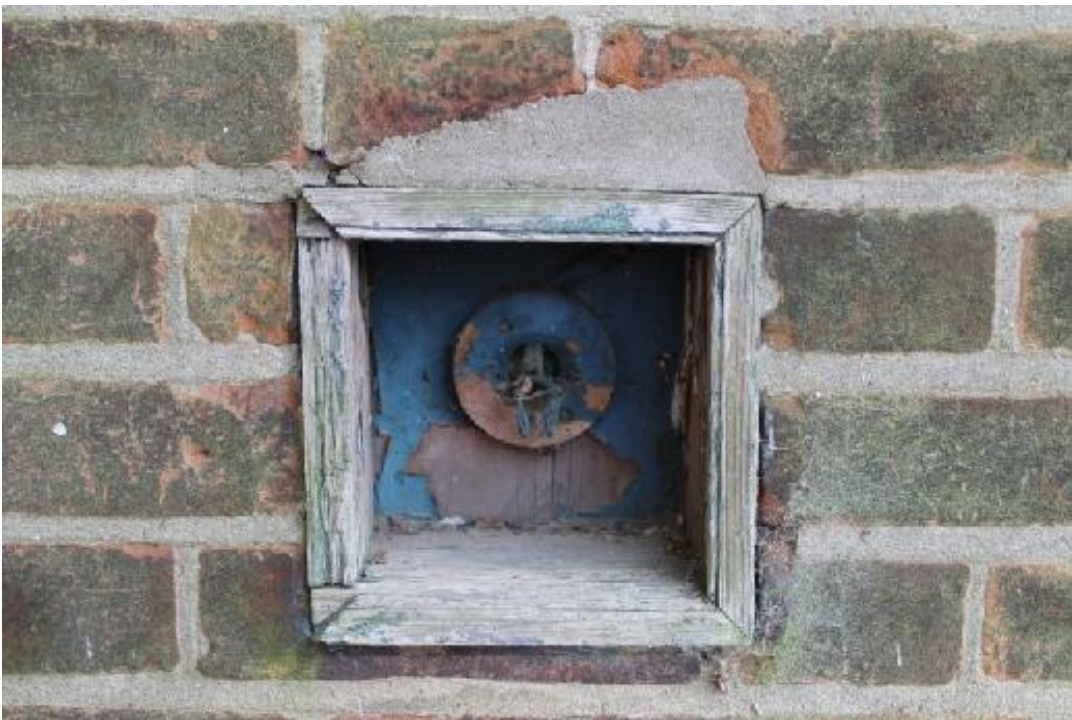
Plate 8 Detail of the wooden housing for electric door bell to the 1904 extension, inserted into the side wall of entrance way i
