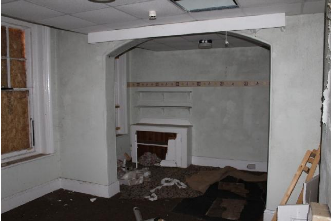
Plate 29 Room 17, the former quarters for Field Officer No.6, showing the repositioned dresser in the sleeping area and the windows without the recessed wooden shutters – view south
