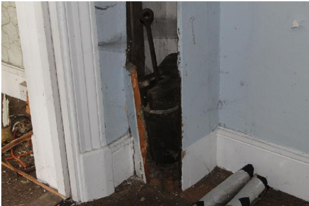
Plate 32 One of the original counter-balances for the food lift, located in the corner of room 18 – view north-east
