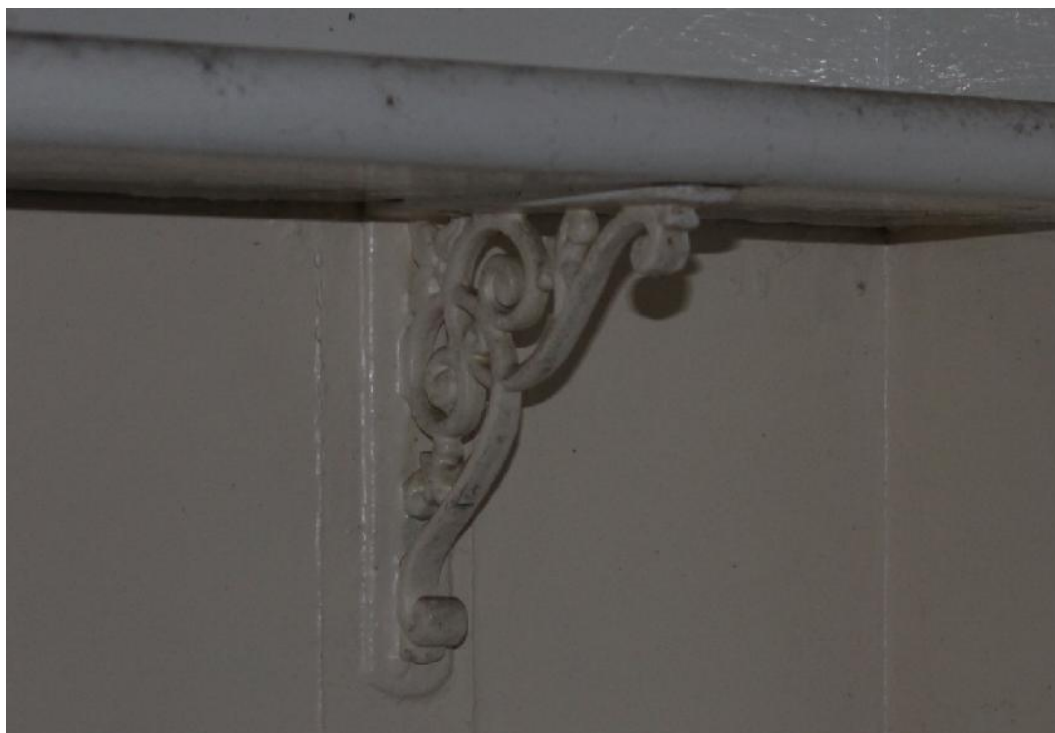
Plate 21 Detail of the ornate shelf brackets common to both the 1876 rooms and the 1904 extensions
