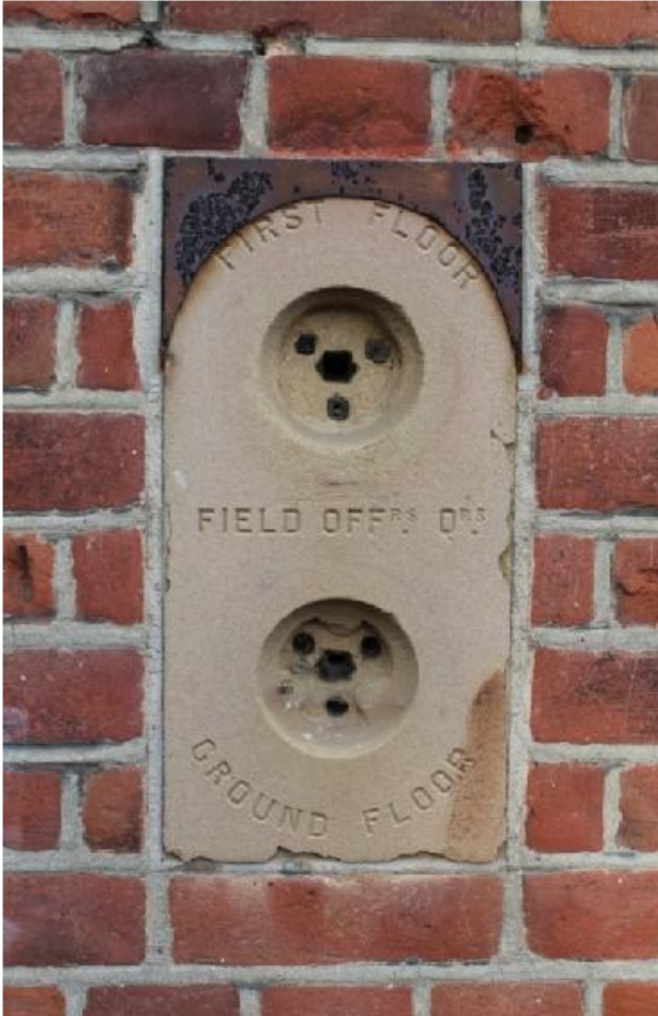
Plate 7 Detail of the sandstone block housing the bell pulls to the Field Officers' Quarters on entrance way i
