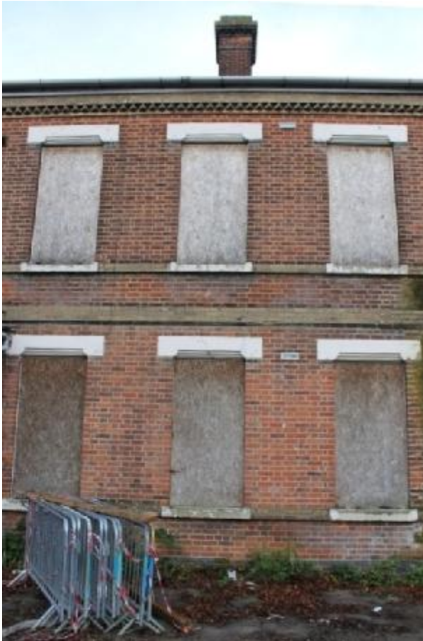
Plate 1 Section of the south-east elevation, showing the windows with their cast lintels and sills and the decorative cornice and string lines of yellow stock brick - view north-west
