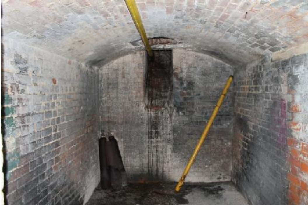
Plate 41 Room 29, the former beer cellar converted to an additional coal store, with a coal chute inserted through the rear wall and the connecting doorway to the wine cellar (in the foreground on the right) bricked in – view north-east
