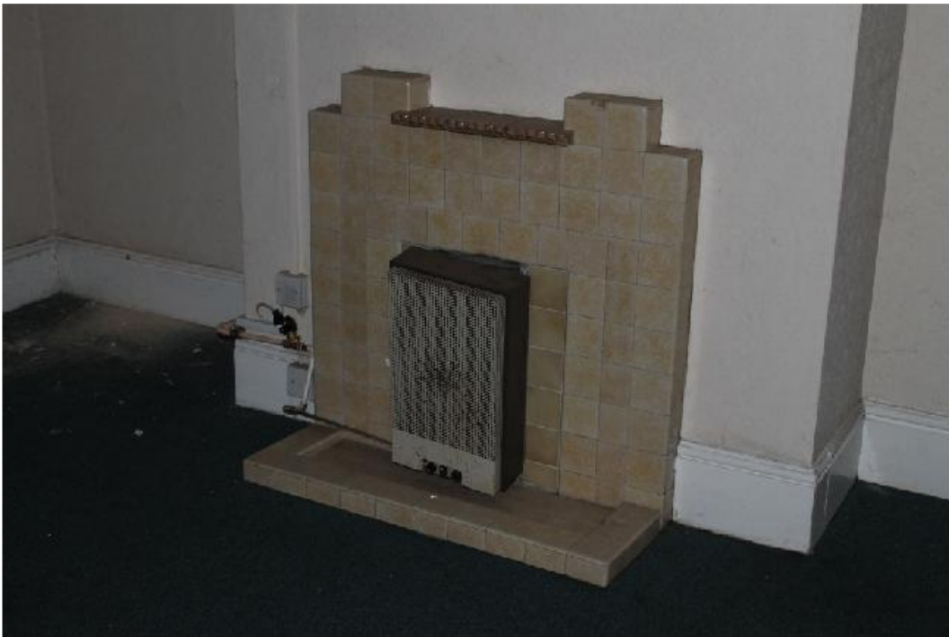
Plate 18 Example of the replacement 1930s Art Deco fireplace with the later gas fire, found in each of the accommodation rooms
