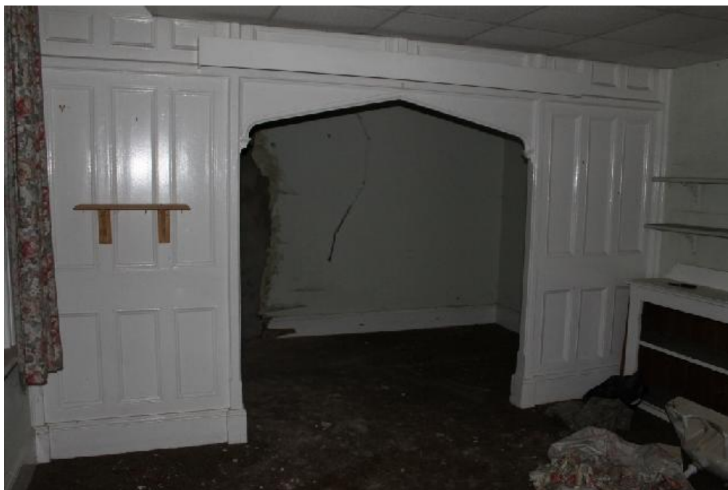
Plate 19 Original wooden partition in room 2 separating the sleeping area from the sitting room – view south-west
