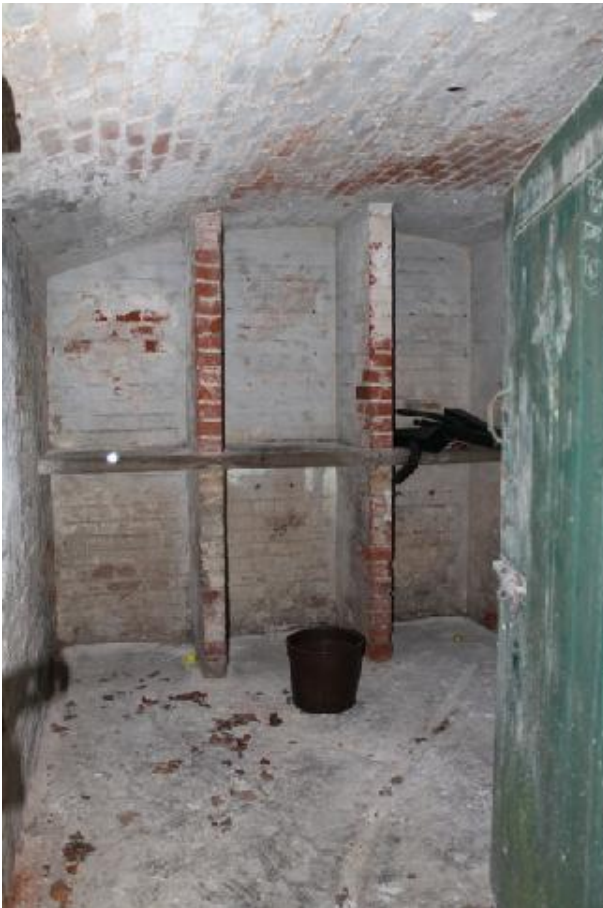
Plate 42 Room 30, the wine cellar viewed through the inserted doorway, with the original sandstone shelves and drainage channel cut into the concrete floor – view north-east
