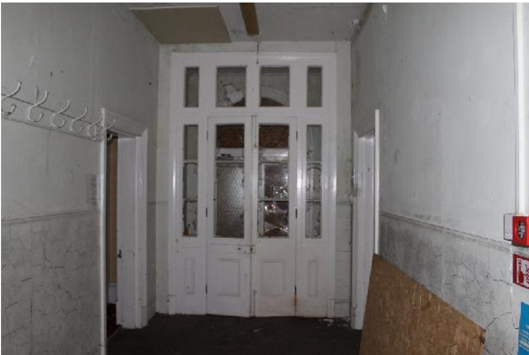
Plate 14 Entrance way ii, showing the original inner and outer doors of the porch and original coat hooks on the left wall - view south-east
