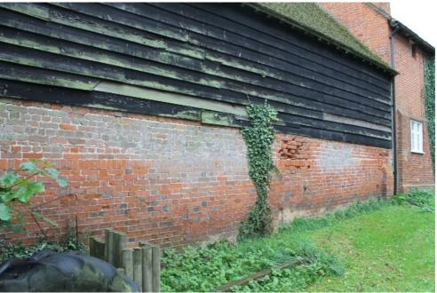
Plate 47 Structure 4 granary/cow house, north-east elevation constructed on the late 18th-century buttressed farmyard wall - view west
