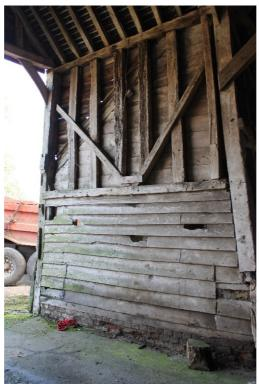
Plate 84 Structure 6 barn, east midstrey with weatherboard to lower register – view east
