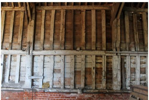
Plate 72 Structure 6 barn, south-west framing of bay 3: the narrow stud in the centre of the upper register has replaced an original window, the diamond-section mortices for the mullions of this can be seen in the underside of the wall plate - view south-west
