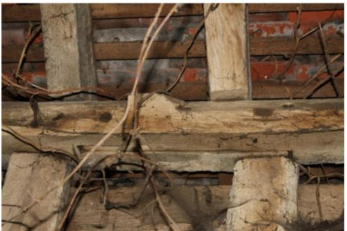
Plate 57 Structure 4 granary, scarf joint in wall plate of north-east frame showing the broached stop of the re-used chamfered beam - view north-east
