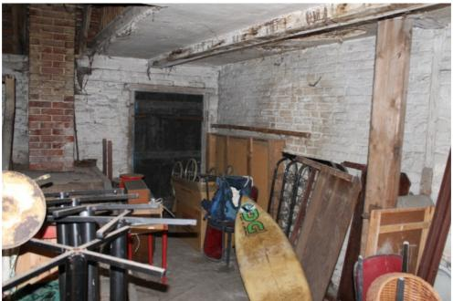
Plate 16 Structure 1/2, interior of FF1 showing the door inserted through one of the blind windows in the north-east wall with the inserted internal chimney stack for the tack room on the left, rising through the landing of the early-mid 18th-century staircase leading to the attic of the main range - view north-east
