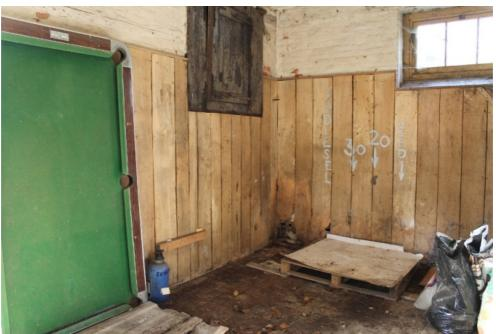
Plate 14 Structure 1/2, interior of stable 2 showing the later plank cladding partially obscuring an original doorway to the left and window to the right - view south-west
