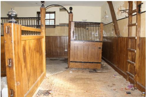
Plate 10 Structure 1/2, interior of stable 1 showing the 19th-century timber and iron stalls with the ladder to the grooms' rooms above on the right along with the chute from the grain bin located on the first floor - view north-east
