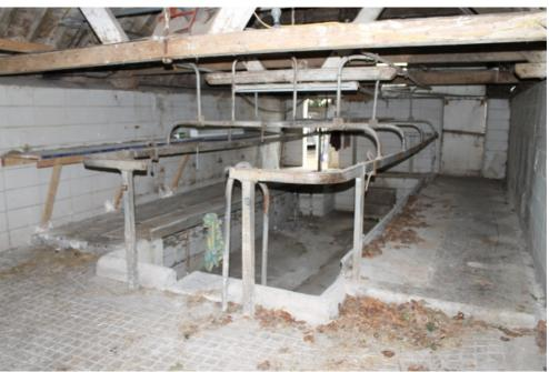
Plate 91 Structure 10 interior of the milking shed, showing the post-1956 'herringbone' parlour layout imported from New Zealand - view northwest
