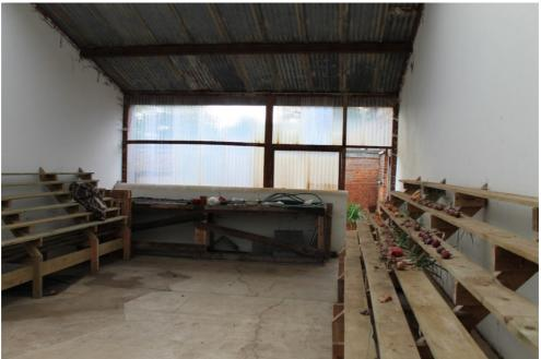
Plate 94 Structure 14 interior of the squash court, showing the original half wall of the south side, the finely grained concrete playing surface and later gardener's shelves - view south
