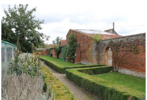
Plate 92 Structure 14 squash court built partially on the east wall of the kitchen garden, showing the buttresses added to spread the load of the building and the archway inserted through the wall providing access to the court – view north-east
