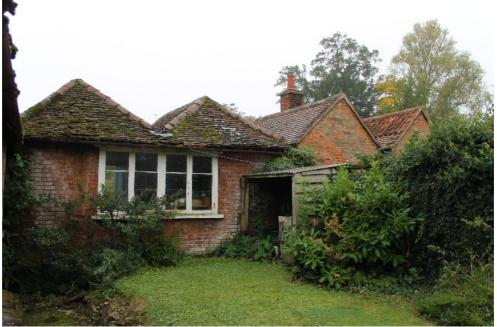
Plate 41 Structure 3a gardener's stores, north-east elevation showing the fully hipped roofs of the potting shed and the gabled ends of the western bays - view south-west
