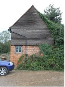
Plate 49 Structure 4, granary/cow house, south-east elevation showing the inserted window above the rebuilt corner - view north-west
