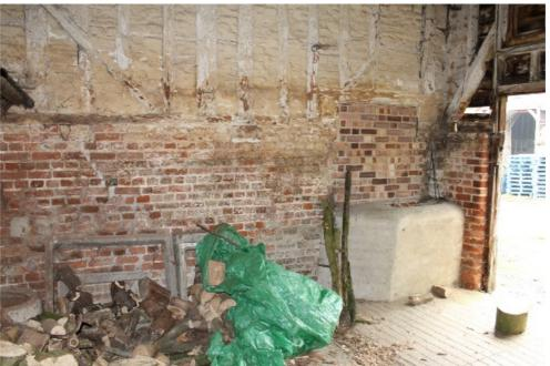
Plate 51 Structure 4 granary/cow house, north-west elevation concealed by the 19th-century infill building showing the raised sill beam of the timber frame and the blocked doorway below - view south-east
