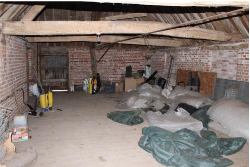
Plate 23 Structure 1/2, interior of FF6 showing the inserted doorway at the far end and the blocked windows in the right-hand wall. The blocked entrance to the first floor of the coach house is just visible to the left of the inserted doorway - view south-west
