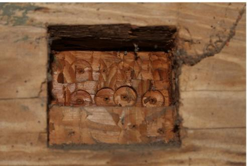
Plate 27 Structure 1/2, detail of exposed mortice in collar beam of attic truss A, showing the drill and chisel technique employed to cut a straight-sided hole - view south-west
