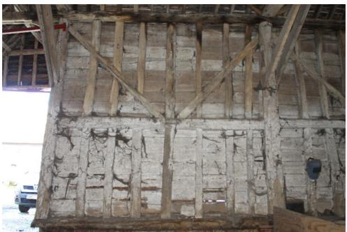
Plate 76 Structure 6 barn, north-east framing of bay 4 with primary bracing to the upper register which indicates a later construction date for this side of the building - view north-east
