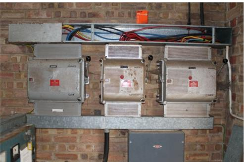
Plate 99 Electrical switches on the dividing wall of the engine room to structure 15; the one for Moor Place is on the left and the others are presumably for the agricultural buildings and the residential dwellings at Home Farm – view east
