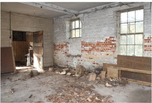
Plate 13 Structure 1/2, interior of garage 1 showing the original window openings with the corbelled lintels and the inserted dividing wall - view south-west
