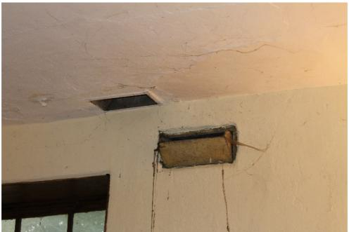
Plate 11 Structure 1/2, interior of stable 1 showing the 19th-century ventilation hopper with the mouth of the shaft for the original Georgian ventilation system in the ceiling to the left - view north
