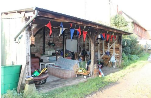
Plate 104 Structure 22 tool shed opposite Farm Cottage, built up against the wall of the laundry drying ground and showing the lightly arched braces to the posts and the low brick plinths and sill beams supporting the posts – view west
