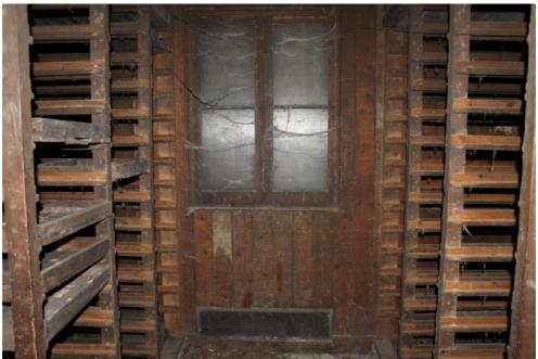
Plate 103 Interior of structure 20, showing one of the windows to the original building and the later tiers of racking for storing trays of fruit in the apple store
