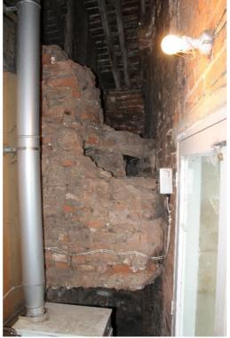
Plate 40 Structure 3 estate office, original brick oven to laundry built up against the kitchen garden wall view east
