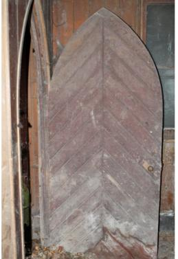
Plate 102 Structure 20, detail of pointed Gothic-style chevron door to interior of the apple store
