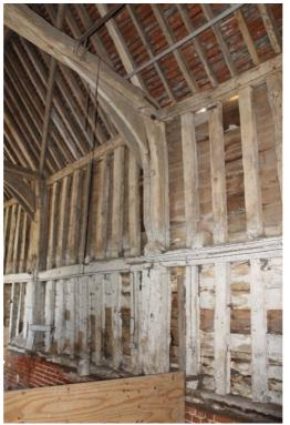
Plate 82 Structure 6 barn, south-west post to truss C with original arched brace to tie beam and later additional straight bracing nailed to the face of post and beam – view south
