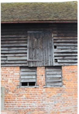
Plate 48 Structure 4, granary/cow house showing inserted pitching door above original louvre windows and the truncated owl door at the top right corner of the door view north-east
