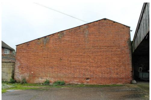
Plate 93 Structure 14 unadorned east elevation of the squash court, showing the long shallow pitch and short steep pitch to the roof - view west
