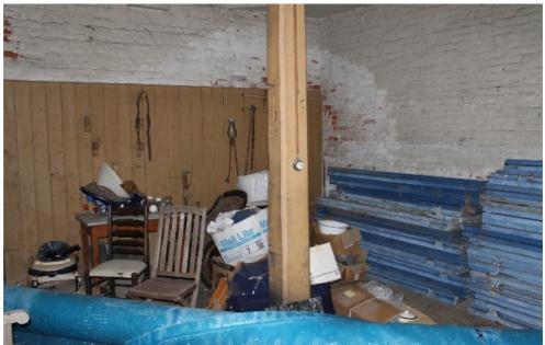
Plate 33 Structure 1/2, interior of garage 2, one of the former carriage stores with plank cladding and harness hooks probably dating to the 19th-century renovations – view west
