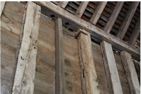
Plate 75 Structure 6 barn, south-west frame of bay 3; diamond-section mortices for window mullions in the underside of the wall plate and mortices for the mid rail forming the sill in the studs to either side of the window: the window interrupts a groove for infill panels in the underside of the wall plate - view south-west
