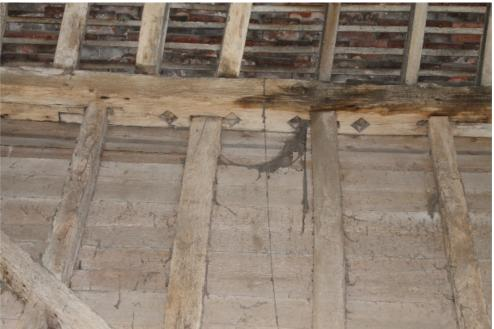
Plate 78 Structure 6 barn, north-east frame of bay 1, diamond-section mortices for window mullions in the underside of the wall plate, which interrupt a groove for infill panels visible in the underside of the wall plate to the right of the frame - view north-east
