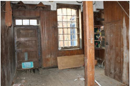
Plate 15 Structure 1/2, interior of the tack room showing the 19th-century plank cladding and the inserted window opening that appears to contain one of the original sash windows. The enclosed staircase leading to the first floor of the main range is to the right - view south-west
