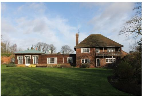
Plate 121 Structure 17 Garden House south elevation showing the single-storey timber extension to the west and the recessed veranda on the first floor – view north
