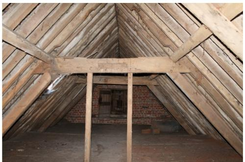
Plate 26 Structure 1/2, interior of the attic to the main range with the chamber housing the clock mechanism to the rear. The principal rafters either side of the collar beam have additional recesses, possibly for a high collar beam - view south-west
