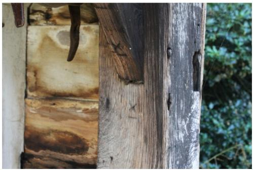
Plate 106 Structure 22, detail of carpenter's marks 'IX' on brace and post - view west
