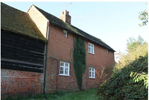
Plate 60 Structure 4a, north-east elevation showing Farm Cottage built upon the early 18th-century buttressed farmyard wall and the 19th-century infill building constructed on the later 18th-century farmyard wall to the left - view south-west
