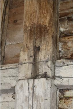
Plate 74 Structure 6 barn, mortice for bridging joist halfway up the post on the south-west side of truss A - view south
