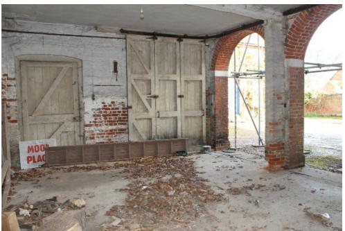
Plate 12 Structure 1/2, interior of garage 1 showing the arches inserted in the 20th century and the Henderson sliding garage doors. The original stable doorway to the carriage arch is to the left - view north-east
