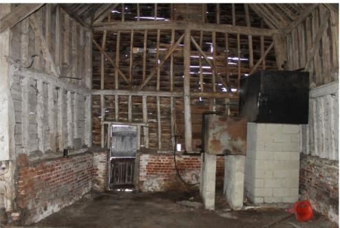
Plate 79 Structure 6 barn, east frame with primary bracing to the upper registers and re-used gable tie - view east
