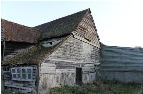
Plate 70 Structure 6 barn, north-west elevation with lean-to 3 to the left, showing the concrete feed troughs and vertical planking indicating an additional (demolished) lean-to - view south-east
