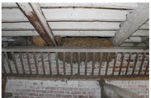
Plate 54 Structure 4 cow house, inserted I-beam and original tie beam carrying the joists of the granary floor - view north-east
