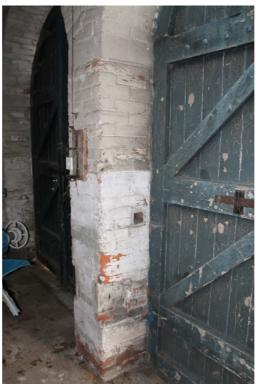
Plate 35 Structure 1/2, interior of garage 2, showing one of the timberlined sockets in the brick pier between the archways, possibly for the original locking bar – view north
