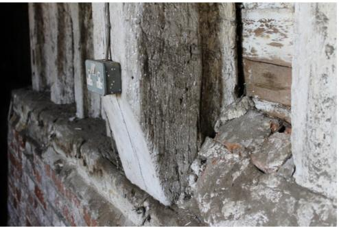
Plate 73 Structure 6 barn, chamfered base to the large-section post on the southwest side of truss A - view south
