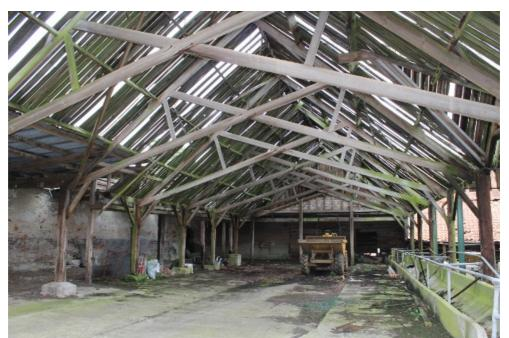
Plate 116 Structure 12 interior of large shed south of barn, showing scissor-braced roof trusses – view north
