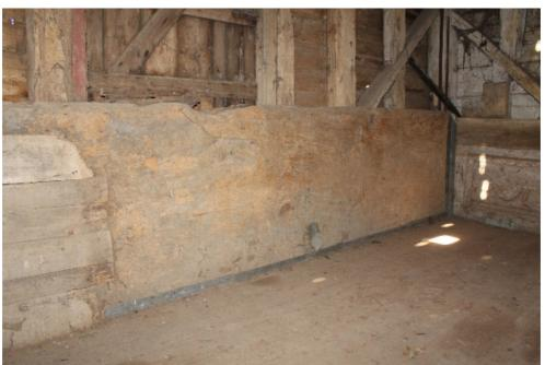
**Plate 80** Structure 6 barn, mezzanine in bay 6 with walls formed from a 1m wide oak plank and doors laid horizontally: the inserted pitching door and primary bracing of the upper register to the north-west frame can be seen behind the mezzanine walls - view north-west
