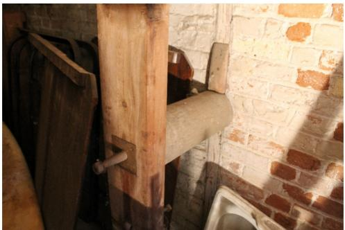
Plate 18 Structure 1/2, winch apparatus in FF1 for hoisting grain sacks up to the first floor through the inserted door in the north-east wall. The early connecting doorway to the first floor of the north range, since blocked, is on the right - view north-east
