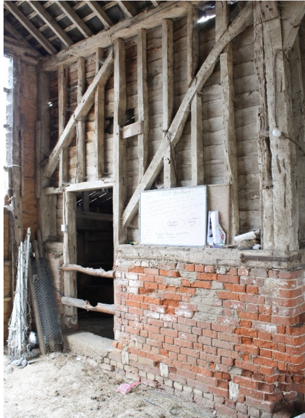
Plate 11 North midstrey with original doorway – view north-west
