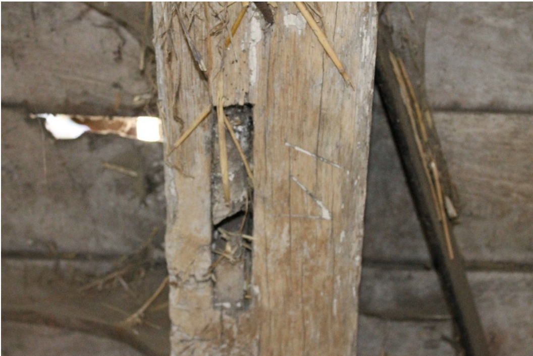
Plate 14 Chiselled carpenter's mark 'VI' on re-used post of truss K - view south-west
