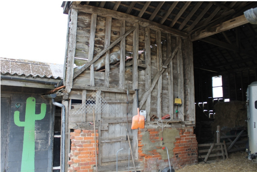
Plate 10 South midstrey with original doorway through brick plinth – view north
