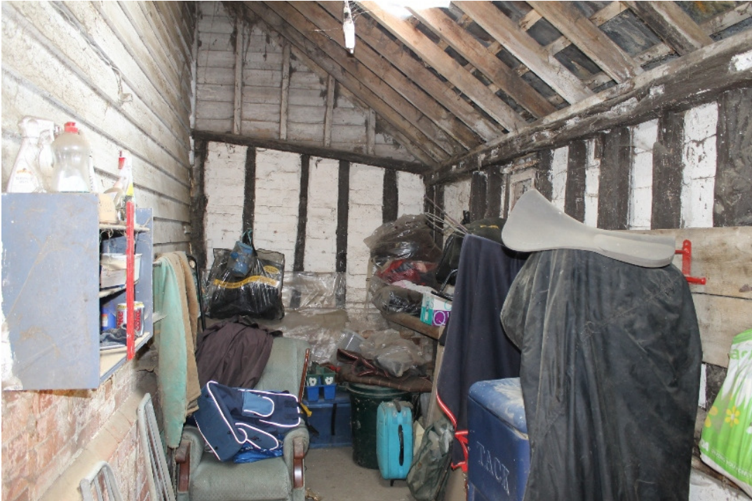
Plate 13 Original lean-to with brick-nogging between studs of end wall – view south-east
