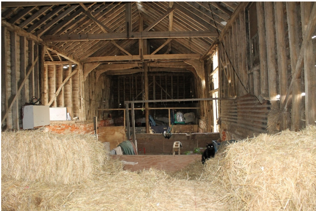
Plate 6 Granary 1b/c – view north-east
