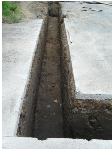
Plate 4 Archive store footings, pit F2. Facing south-west.
