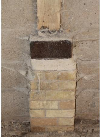
Plate 14 Detail of brick and iron plinth for timber post of shelter shed 8
