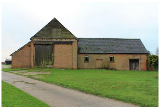
Plate 4 Straw barn 2, note the sliding door and ornate cornice (with shed 1 to the right) - view south-west
