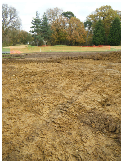
Plate 2: a land-drainage pipe trench, view north-east.
