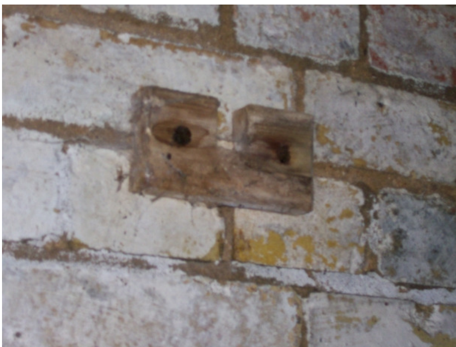
Plate 8 West shelter, surviving original bracket for curtain across toilet recess - view north.
