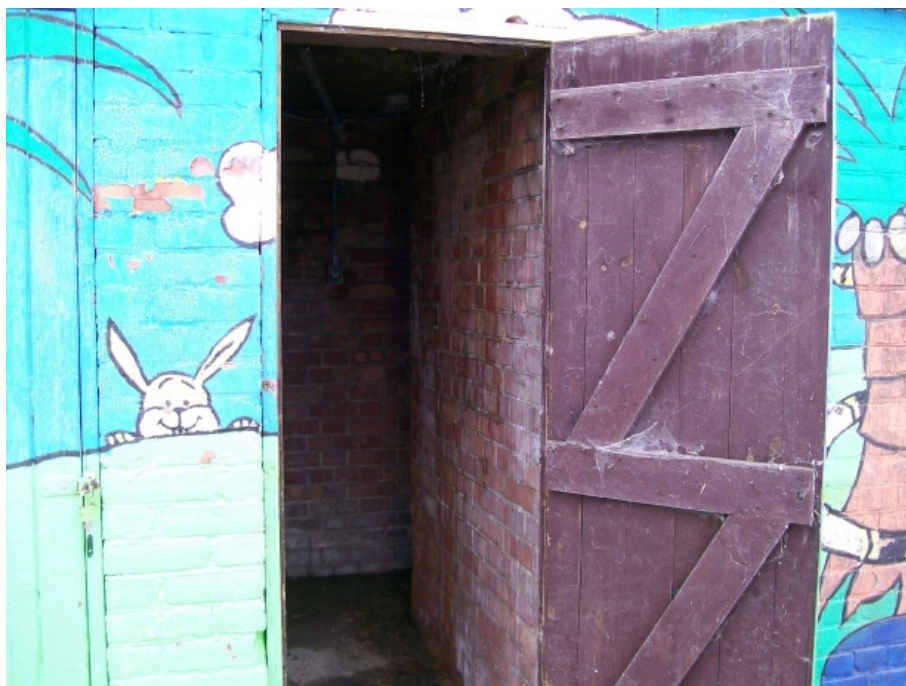
Plate 2 East shelter entrance with blast wall to the right - view north.
