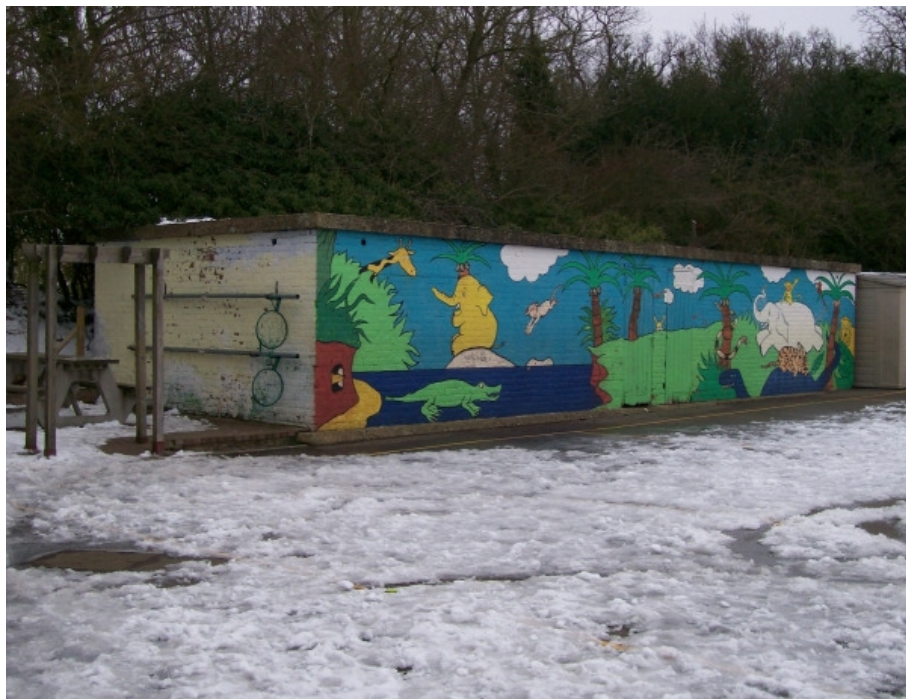
Plate 1 Air-raid shelter - view north-east.
