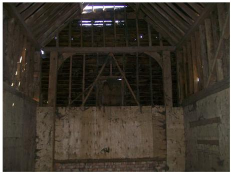
**Plate 3** Building A, blocked doorway to south midstrey with original doorposts and hanging knee braces.
