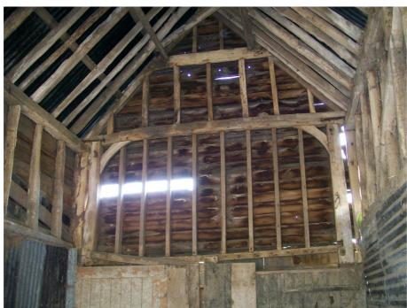
Plate 8 Building B, blocked doorway to midstrey with hanging knee braces and strengthening iron staples.
