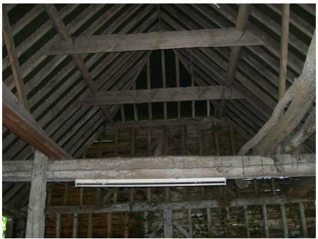
Plate 18 Building G, interior showing nailed tie beam support and collar-clasped purlins.
