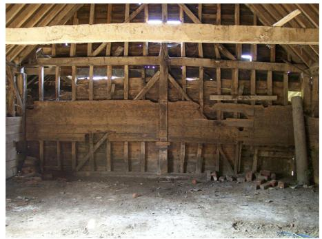
Plate 14 Building E, interior showing plank cladding on south wall.
