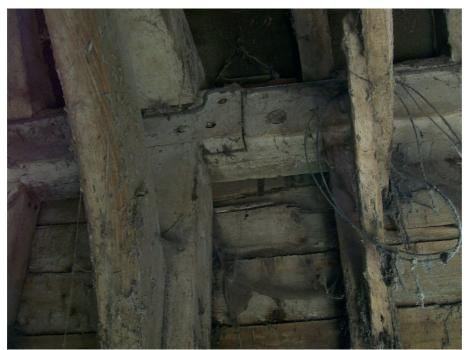
Plate 13 Building E, detail of wall plate scarf joint.
