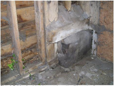
Plate 4 Building A, original doorpost clasped by sill beam, bay 3.
