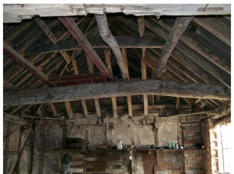
Plate 16 Building F south end, showing cambered tie beam, infilled timber-framing and original hipped roof timbers.
