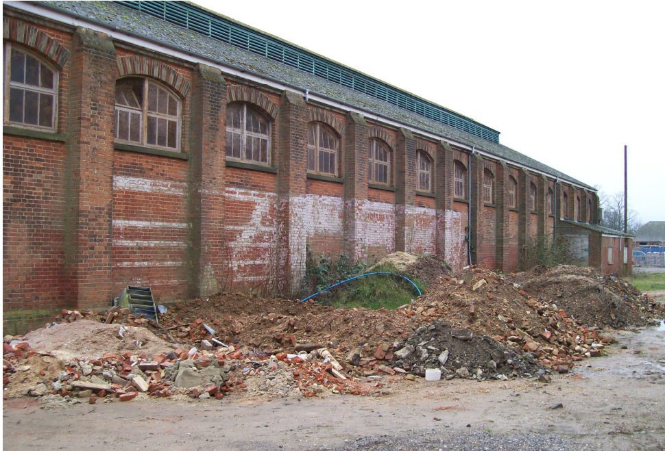
Plate 5. North-west wall showing additional structure.
