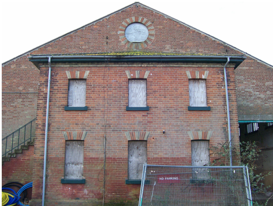
Plate 1. North-east end, three window range annexe with oculus above.
