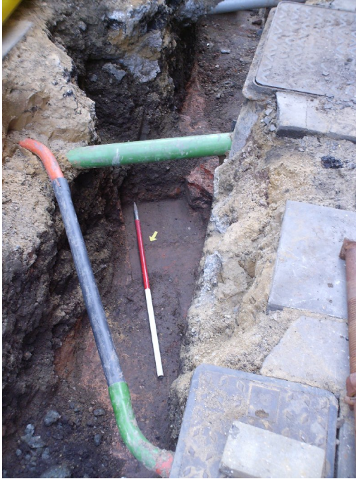
Plate 3 Roman drain F12, viewed from the north-west.
