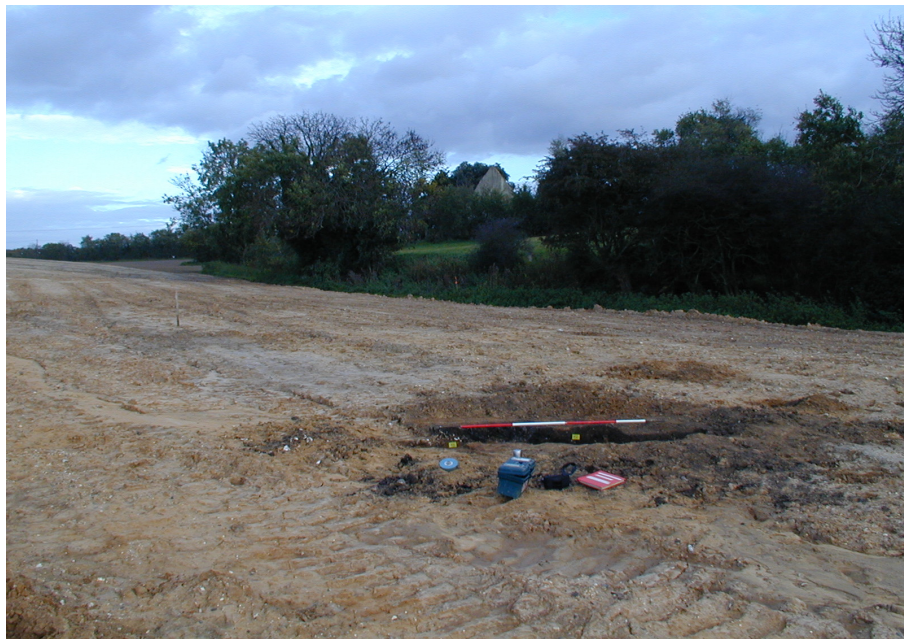
Plate 2 Area 2: general location, looking east.
